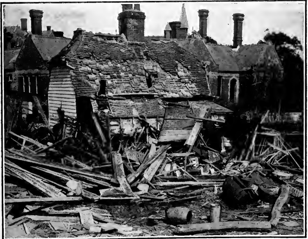
AT MALDON, ESSEX. A demolished workshop in Spital Road.
