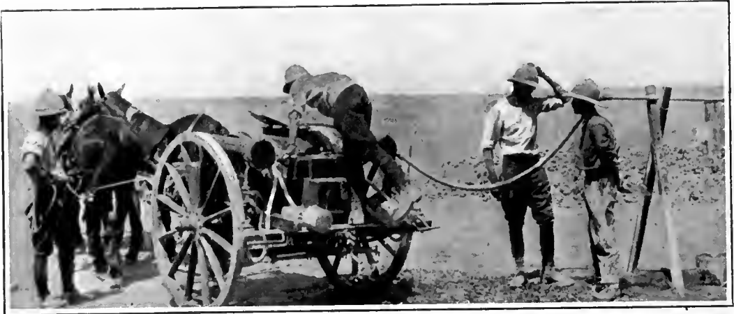
FILLING A WATER CART FROM A NEWLY-SUNK WELL.
