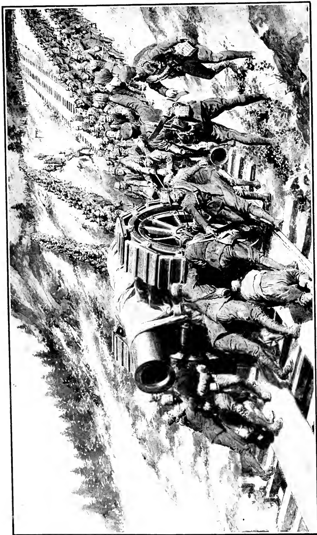
ITALIAN SOLDIERS HAULING A HEAVY ITALIAN MORTAR ABOVE THE MOUNTAIN SLOPES. Getting over difficulties in the high Alps. The road over which the gun travelled was constructed of timbers laid crosswise, after the style of railway sleepers. On these timbers parallel planking was placed to take the mortar wheels.
