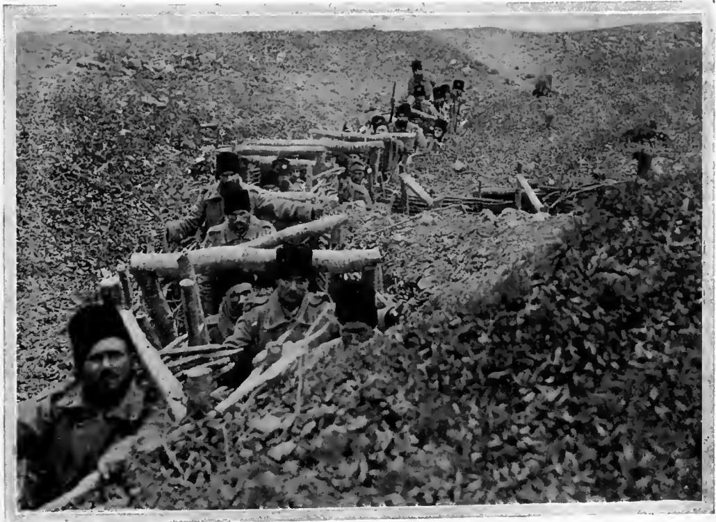
A COMMUNICATION TRENCH.
