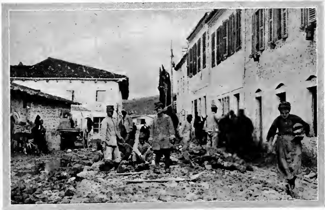
ITALIAN RESERVISTS REPAIRING ROADS IN VALONA.
