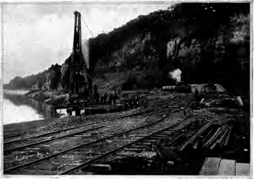
THE BEGINNINGS OF A SHIPYARD: THE SITE AND A TEMPORARY WHARF.
