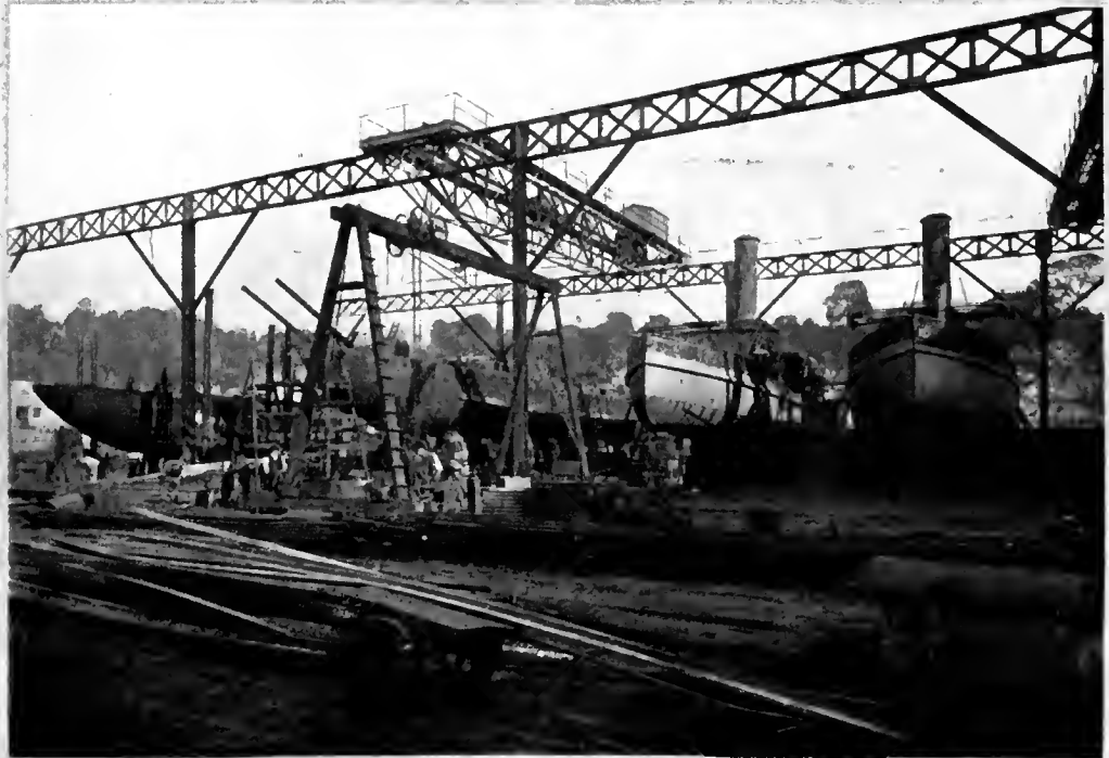
THE OLD SLIPS. INSET: AN EXCAVATOR.
