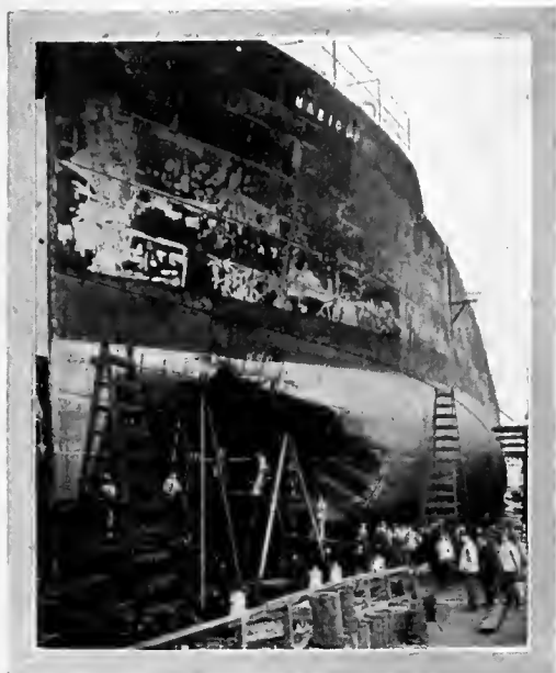
REPAIRING A SHIP DAMAGED BY A MINE.
