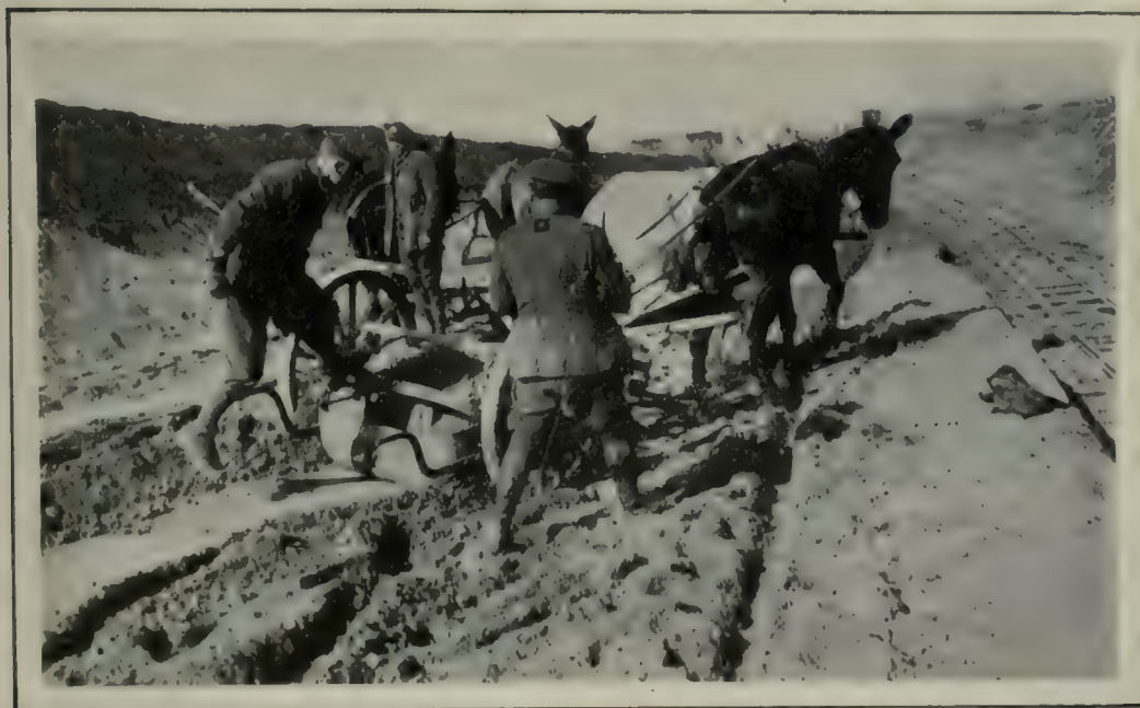
ROAD-MAKING IN THE RECONQUERED AREA: THE SCOOPER AT WORK.
