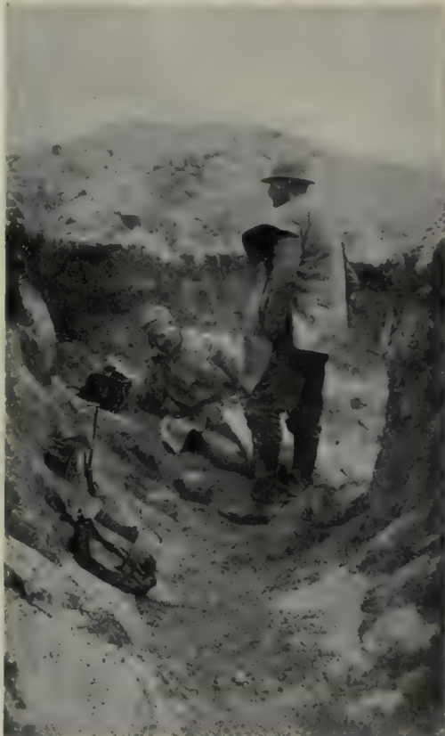
ON THE CHEMIN DES DAMES: A FRENCH TELEPHONE STATION.
