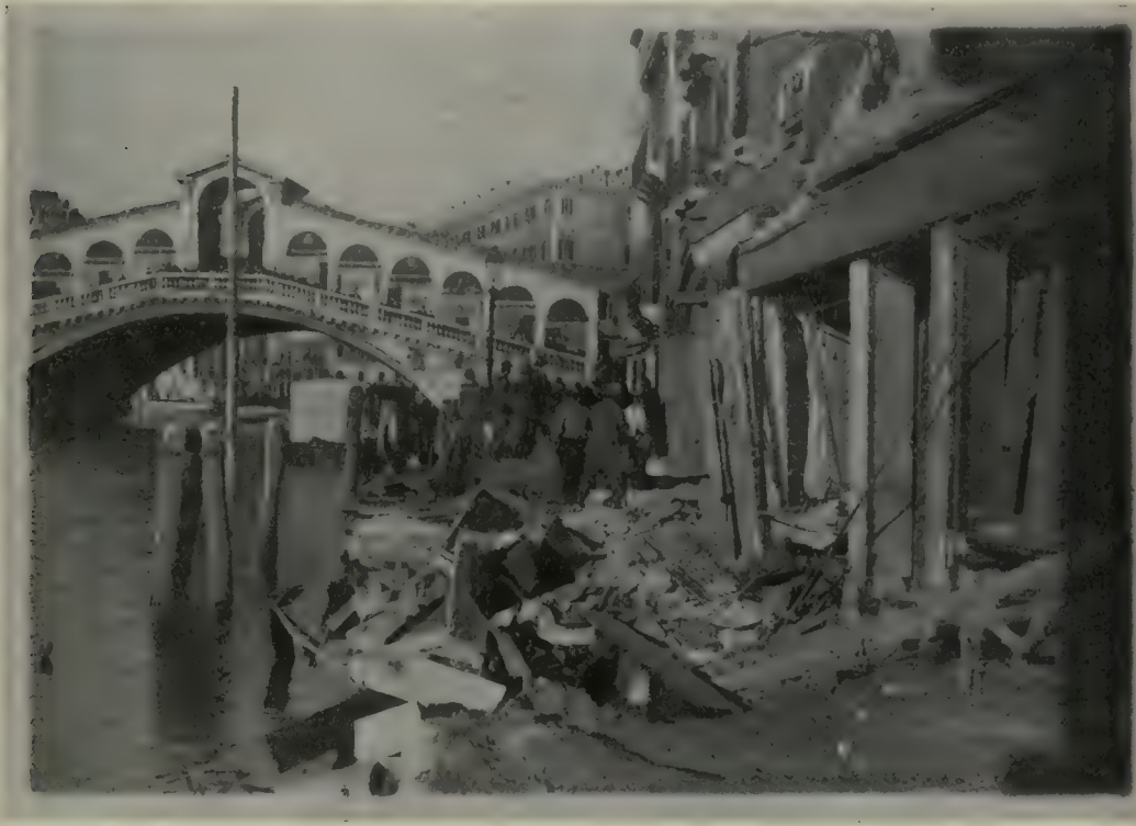
BOMBED BUILDINGS ADJOINING THE RIALTO BRIDGE.
