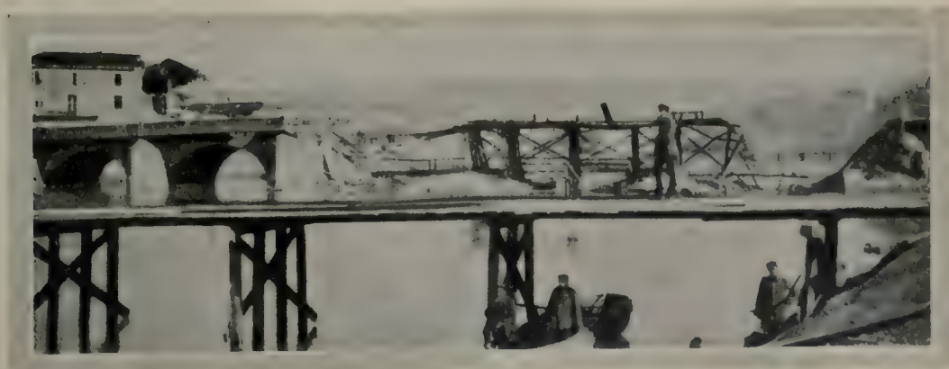
ST. MIHIEL: A TEMPORARY BRIDGE ACROSS THE MEUSE.
