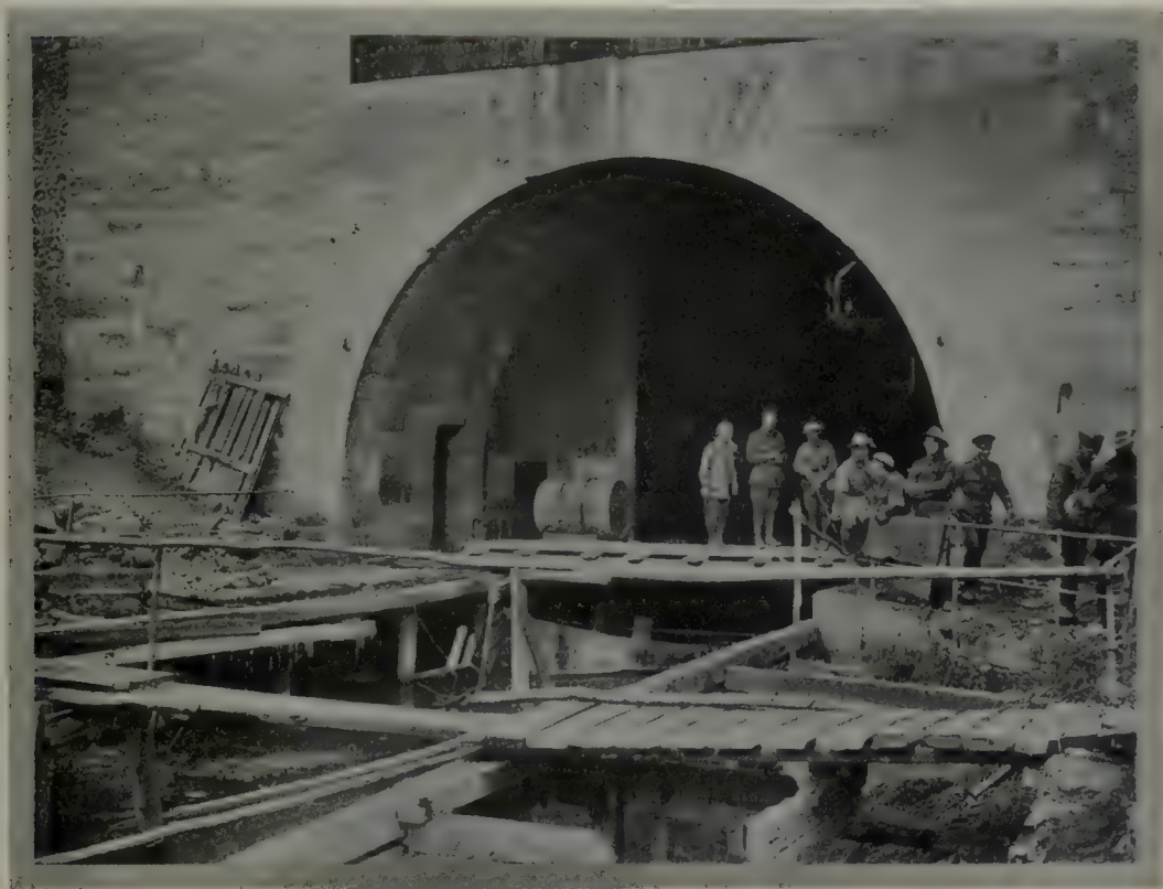
TUNNEL ON THE ST. QUENTIN CANAL.
