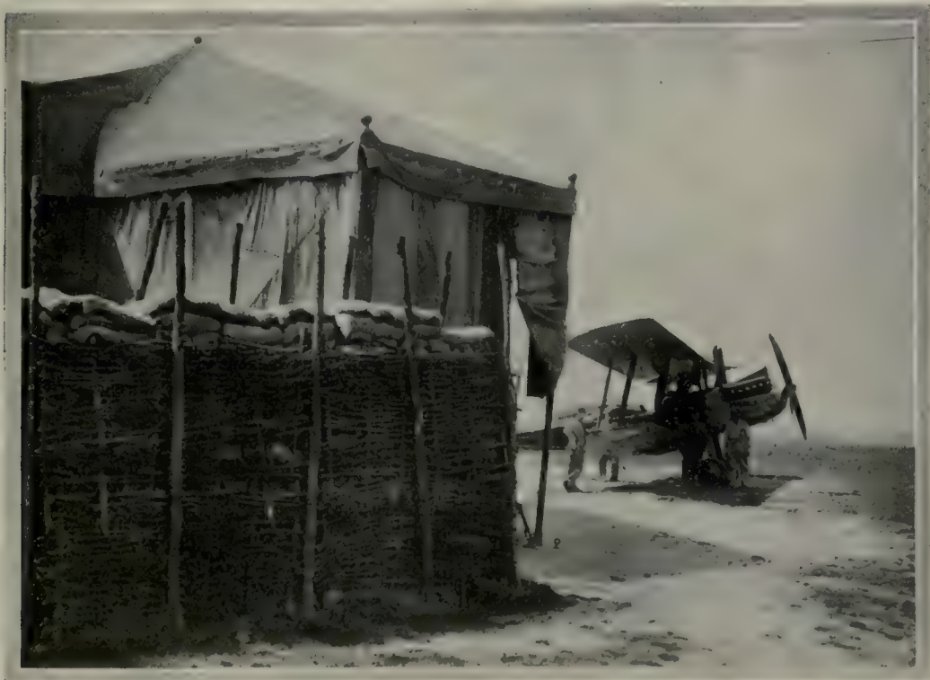
SAND-BAG PROTECTION FOR AEROPLANES.
