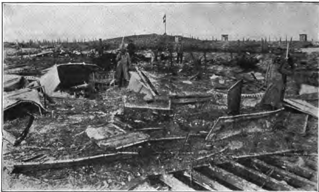
GROUND SURROUNDING ONE OF THE LIÈGE FORTS. Showing shattered armour plate.
