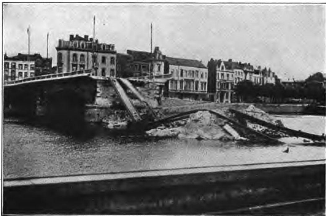
ANOTHER VIEW OF THE RUINED BRIDGE.
