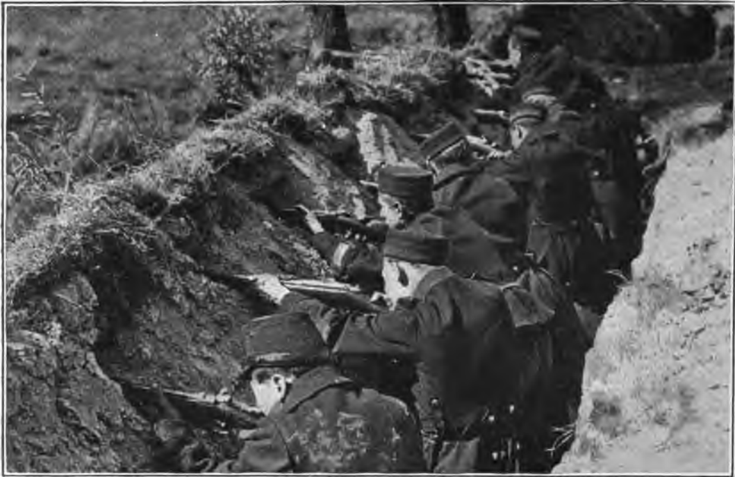
INSIDE A BELGIAN TRENCH.
