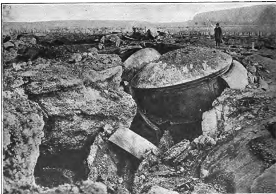
ONE OF THE FORTS AT LIÈGE AFTER BOMBARDMENT. Showing damage caused by German siege guns.
