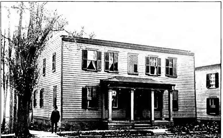
1. Hyde Hall. 2. Pomeroy Place. 3. Masonic Hall.
