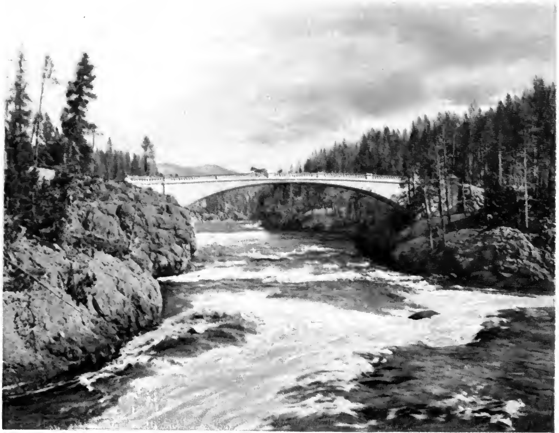
Bridge above The Rapids
