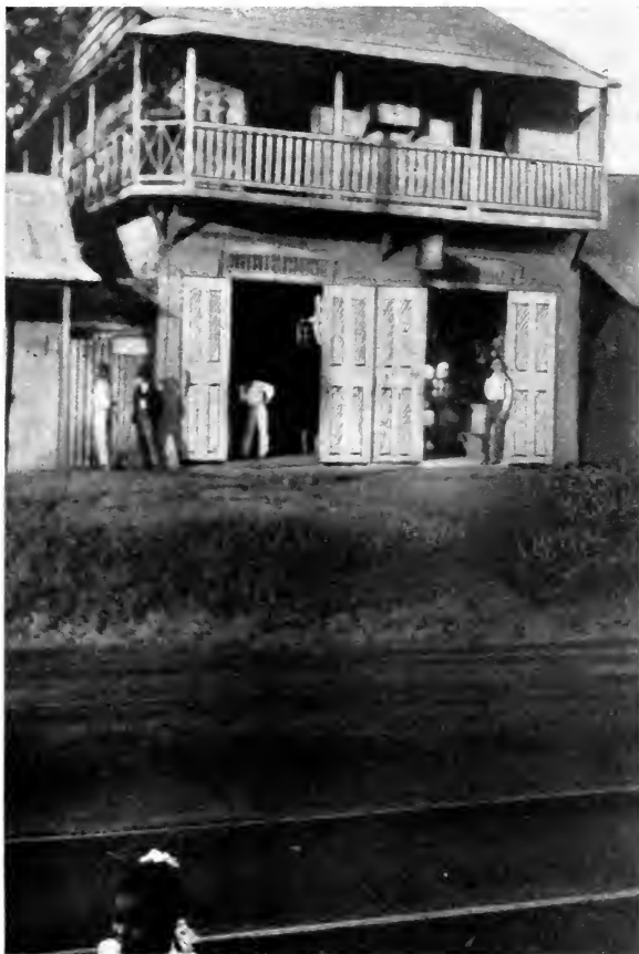
COMBINATION STORE AND RESIDENCE AT BOCAS DEL TORO
