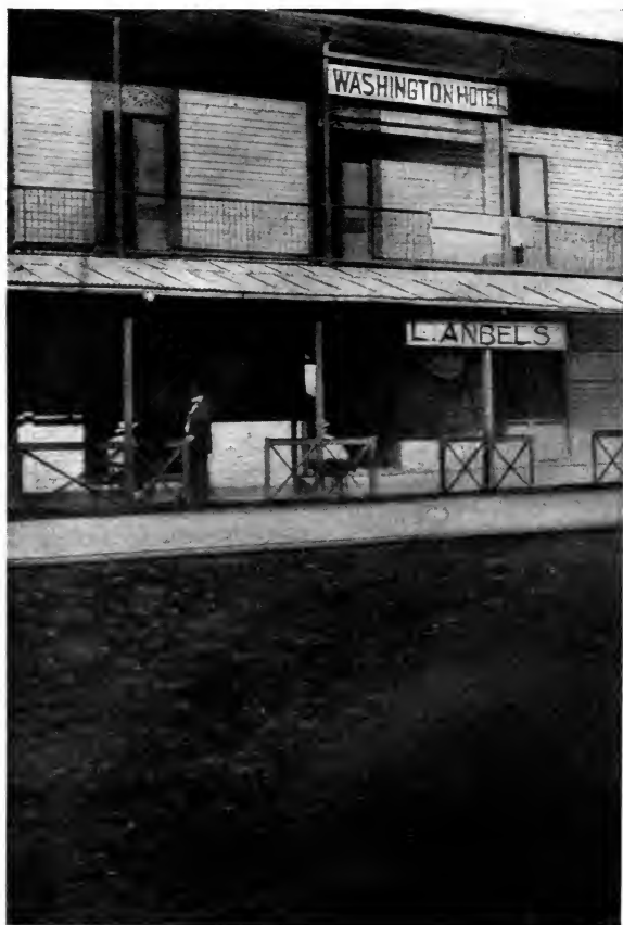
WASHINGTON HOTEL, STREET FRONT, COLÓN
