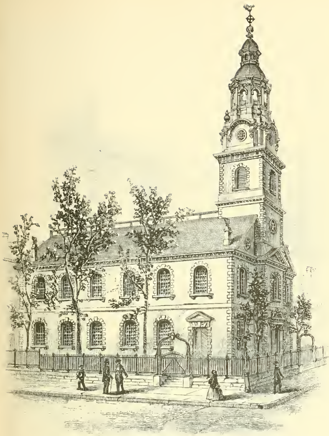
NORTH DUTCH CHURCH, FULTON STREET
