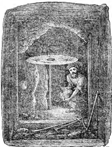
INVERTED COLUMN FOUND IN UNDERGROUND PASSAGE.
