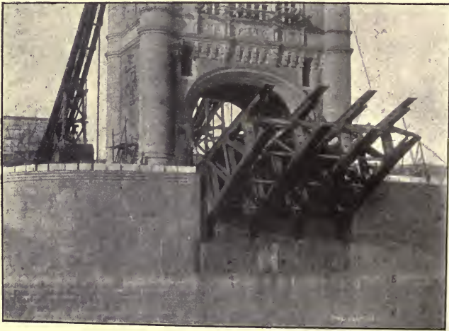
FIG. 36. MOVING GIRDERS IN PROGRESS.
