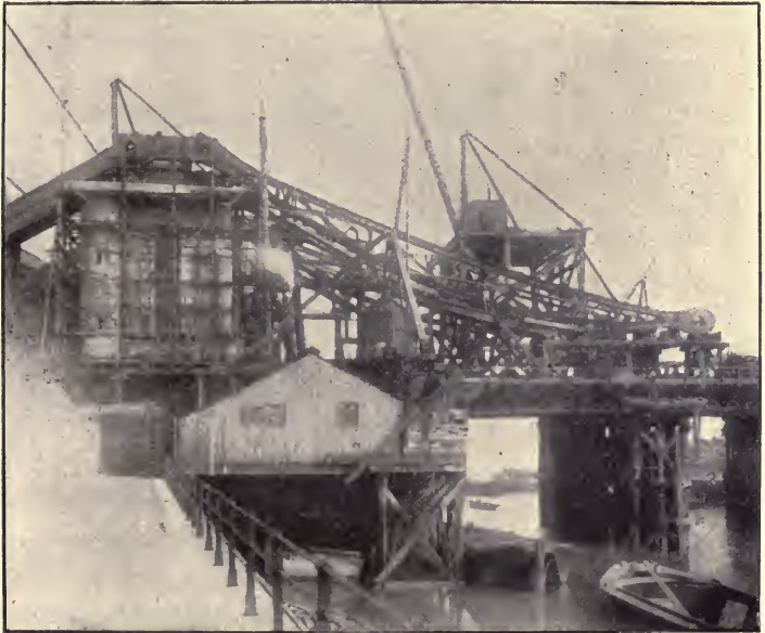
FIG. 33. PROGRESS OF ERECTION OF MAIN CHAINS. SHORT SEGMENT.]
