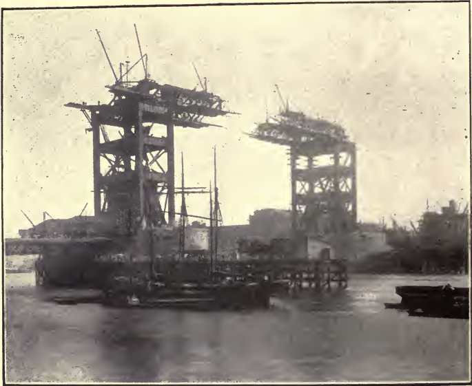
FIG. 32. PROGRESS OF HIGH-LEVEL BRIDGES.
