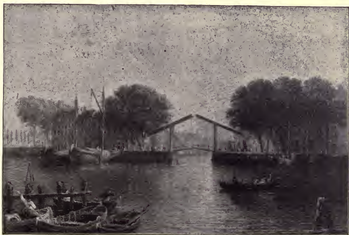
FIG. 9. BASCULE BRIDGE ACROSS A DUTCH CANAL.
