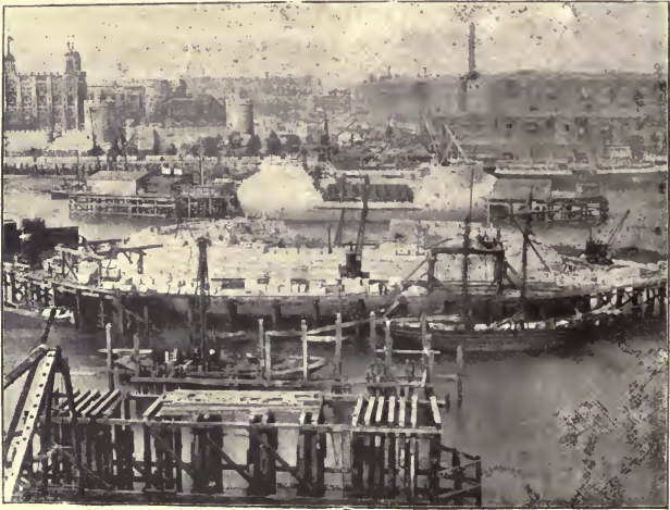
FIG. 26. VIEW OF THE FOUNDATIONS IN PROGRESS.
