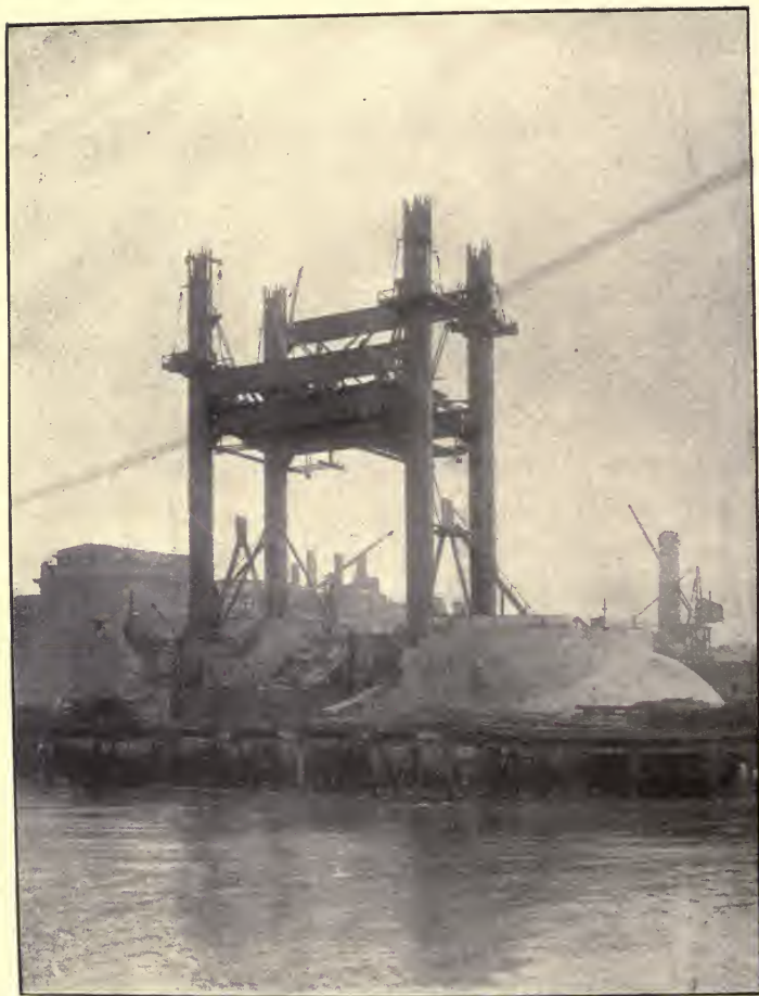
FIG. 31. PROGRESS OF TOWER ON PIER IN RIVER.
