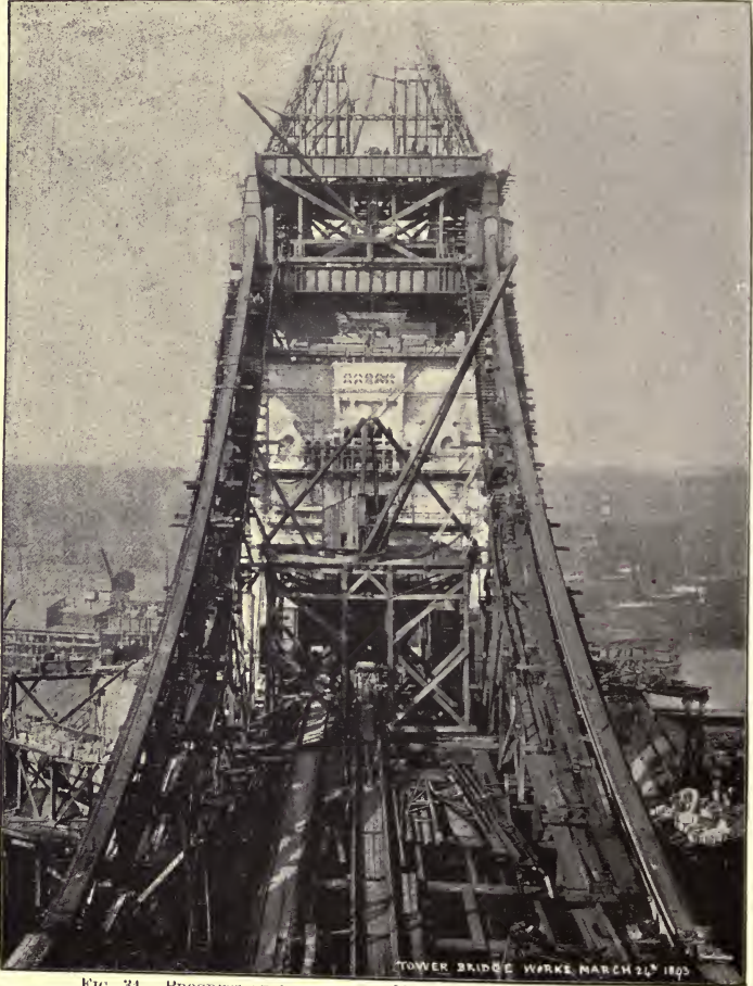
FIG. 34. PROGRESS OF ERECTION OF MAIN CHAINS. LONG SEGMENT.
