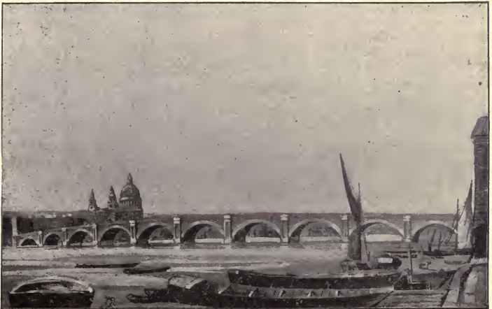
FIG. 5. OLD BLACKFRIARS BRIDGE.
