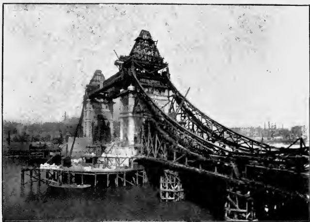
FIG. 35. PROGRESS OF ERECTION OF MAIN CHAINS. GENERAL VIEW.
