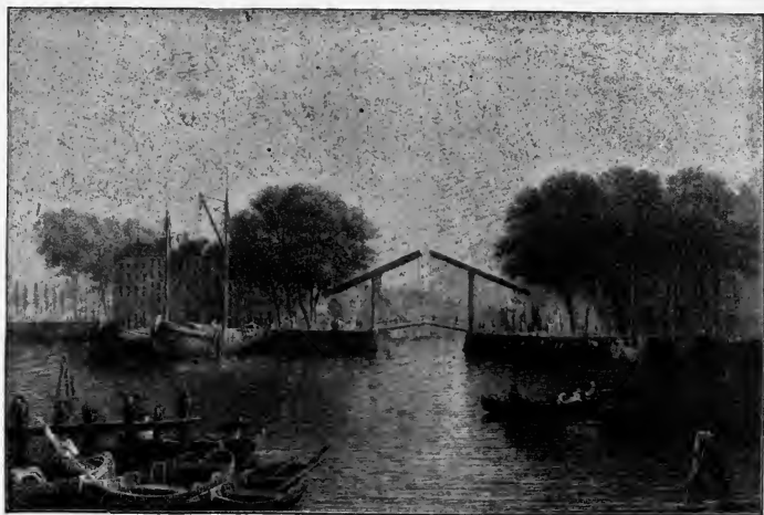
FIG. 9. BASCULE BRIDGE ACROSS A DUTCH CANAL.
