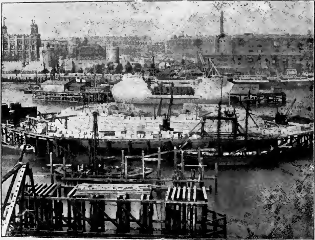
FIG. 26. VIEW OF THE FOUNDATIONS IN PROGRESS.
