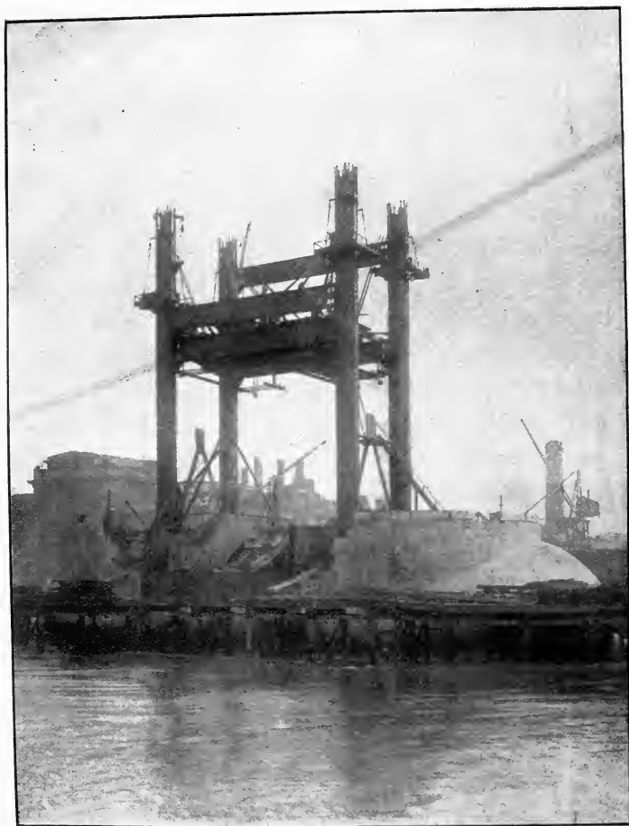
FIG. 31. PROGRESS OF TOWER ON PIER IN RIVER.
