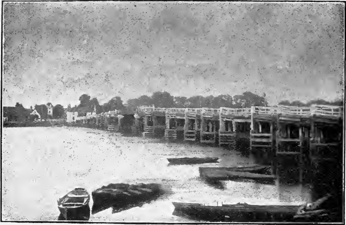
FIG 1. OLD PUTNEY BRIDGE.
