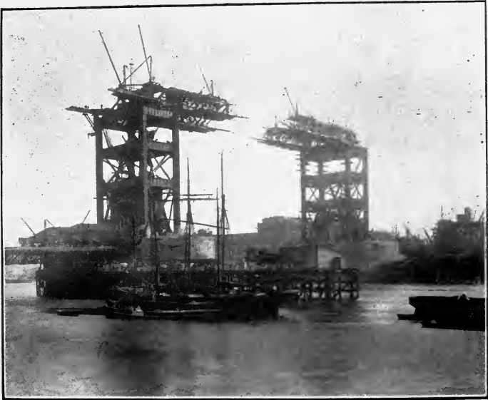
FIG. 32. PROGRESS OF HIGH LEVEL BRIDGES.
