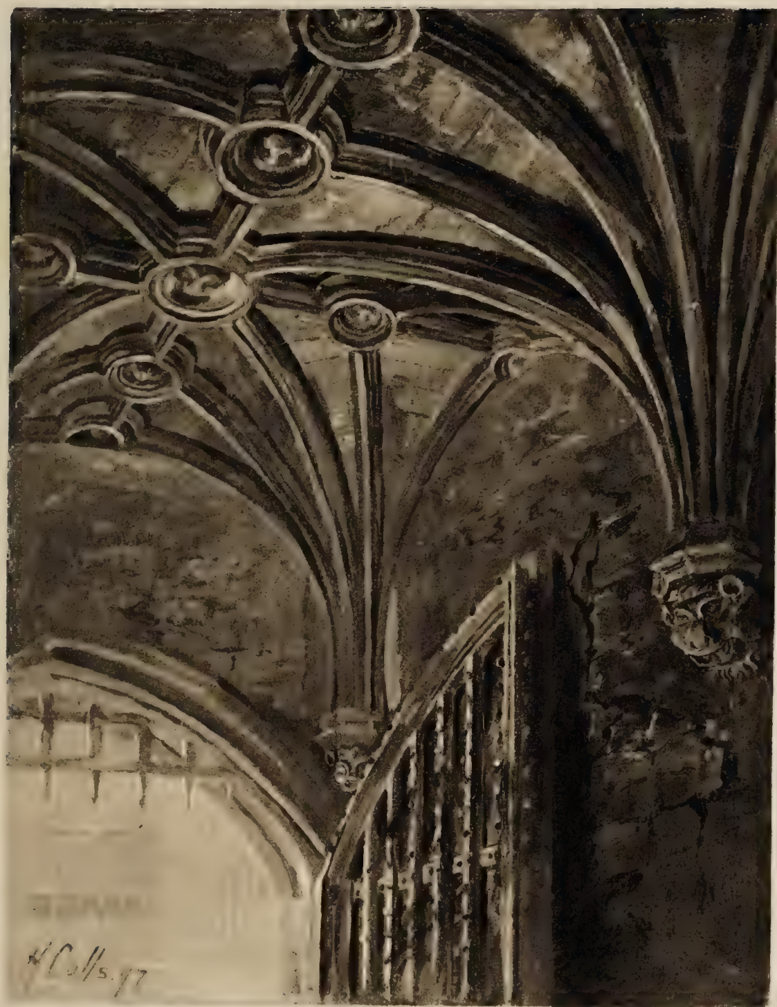
Groining in Ceiling of the Bloody Tower.
