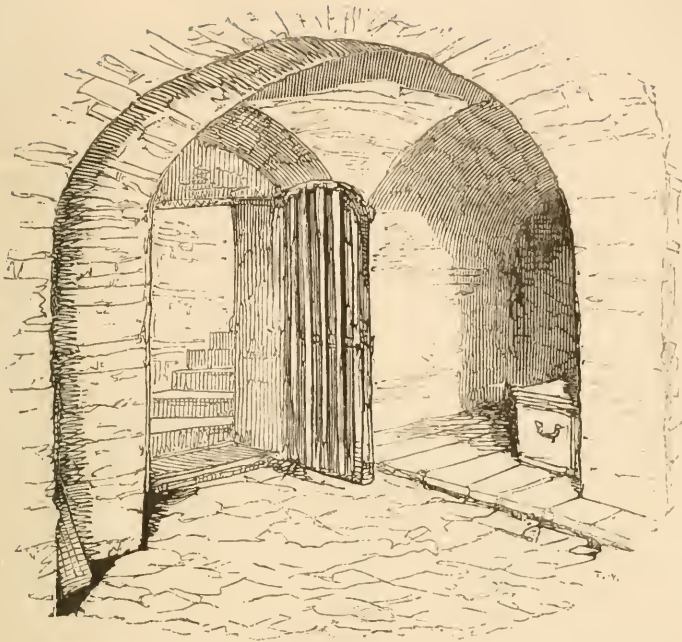
BASEMENT CHAMBER IN THE FLINT TOWER.
