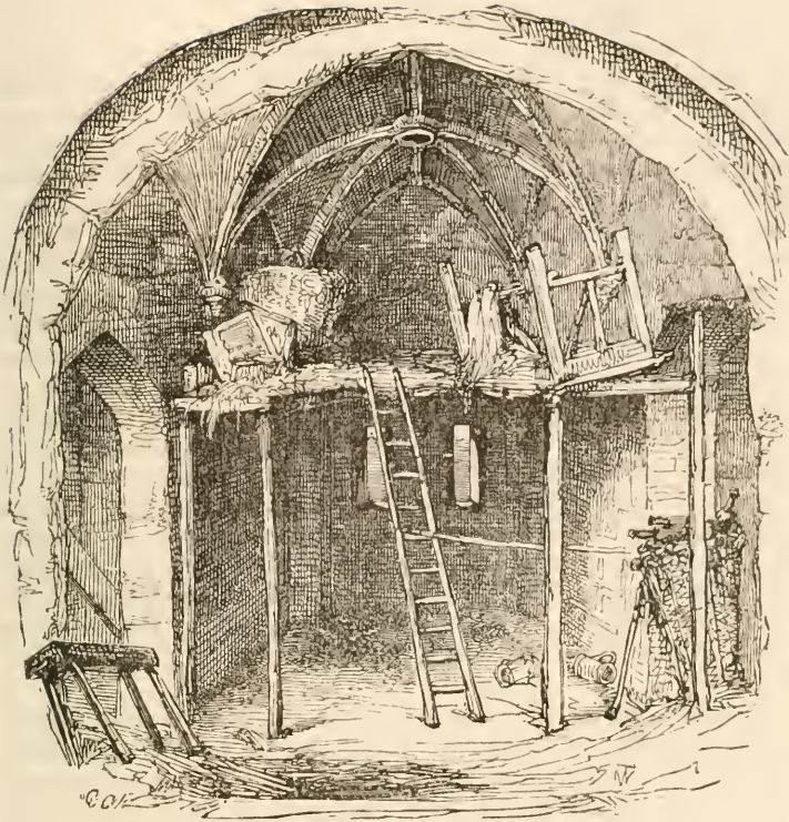
INTERIOR OF THE CRADLE TOWER.
