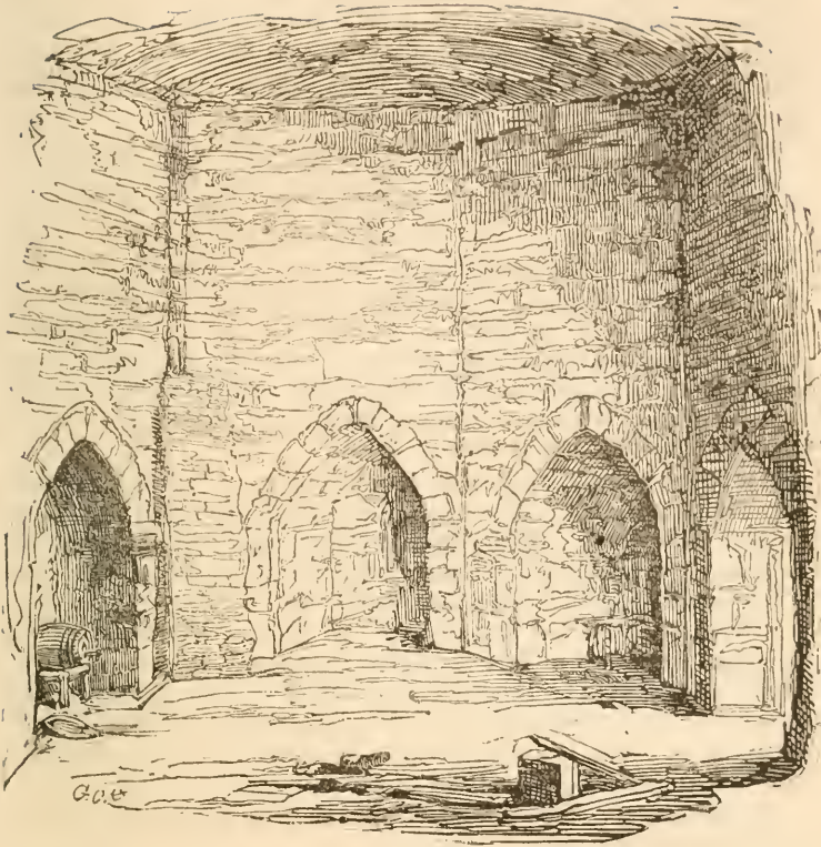
BASEMENT CHAMBER IN THE SALT TOWER.
