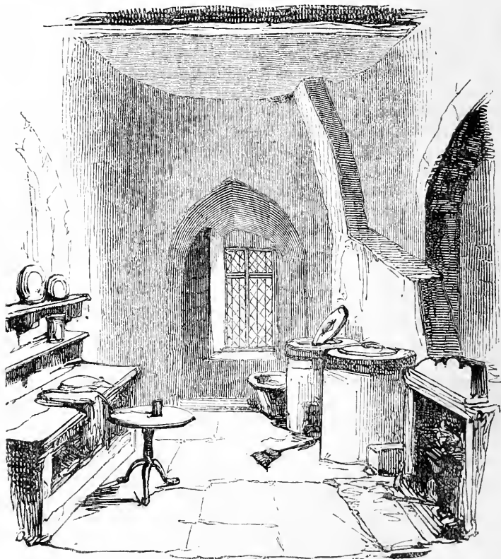
LOWER CHAMBER IN THE CONSTABLE TOWER.
