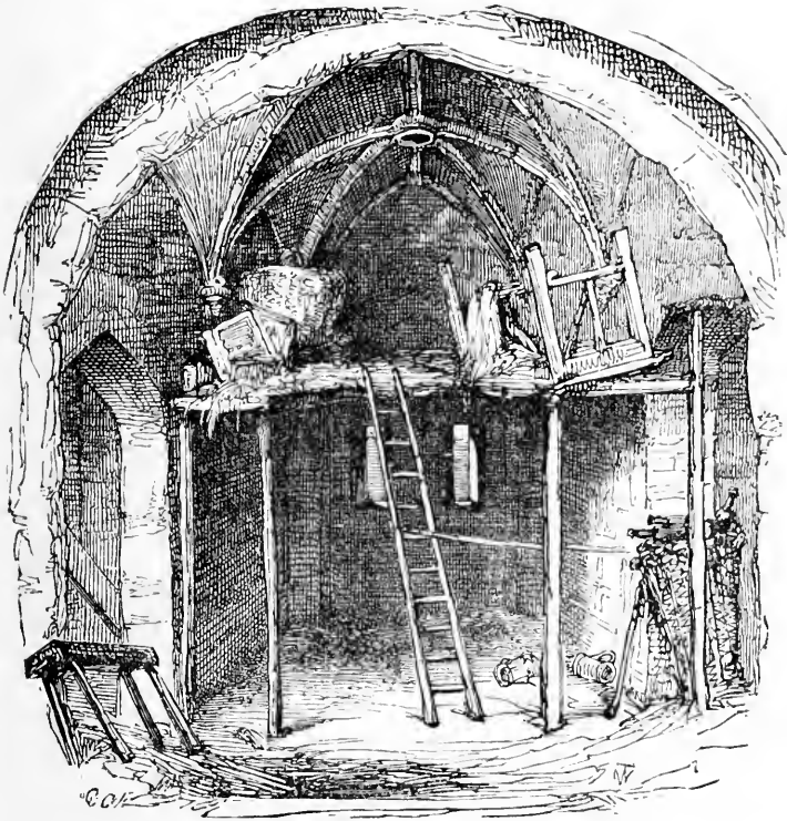
INTERIOR OF THE CRADLE TOWER.
