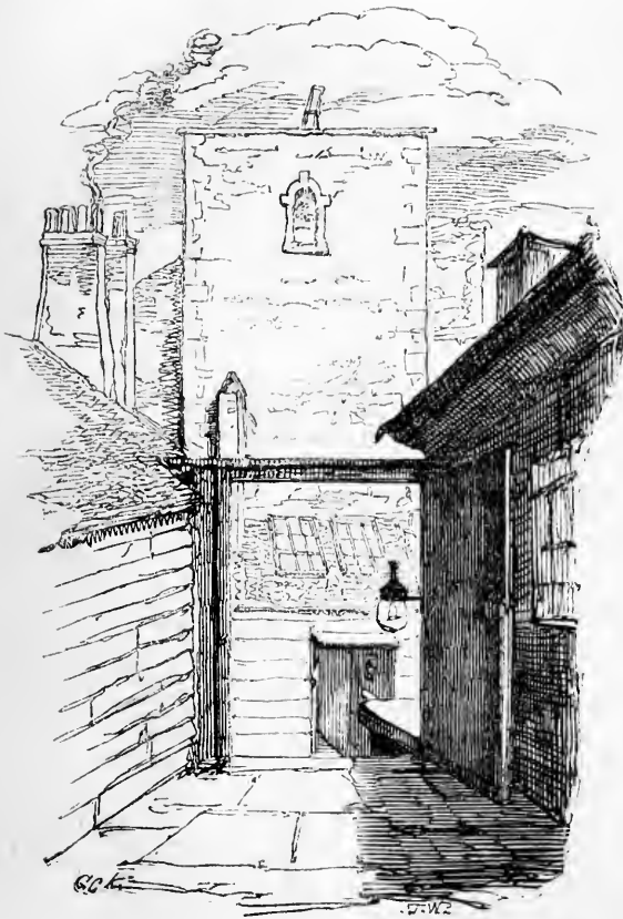
NORTH VIEW OF THE SALT TOWER.
