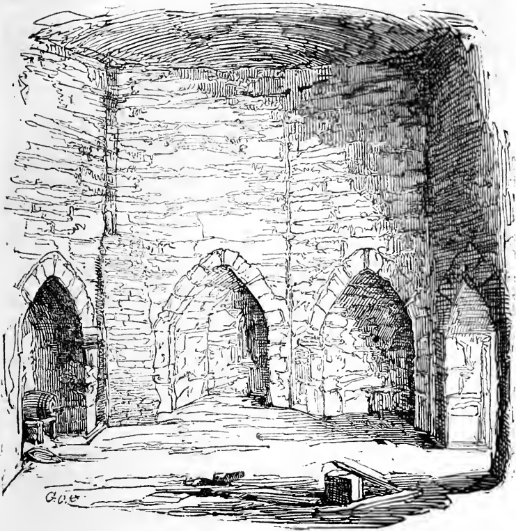
BASEMENT CHAMBER IN THE SALT TOWER.
