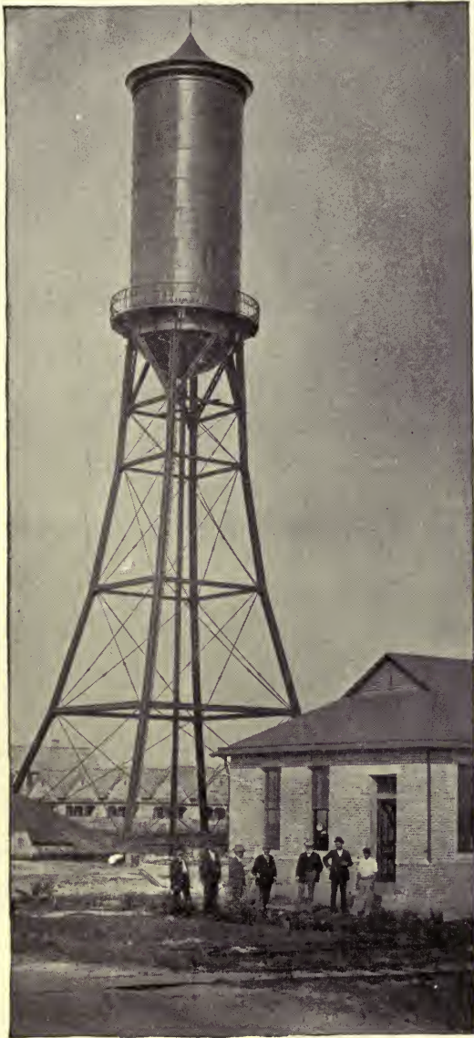
TOWER AND TANK, WEST TAMPA, FLA.
