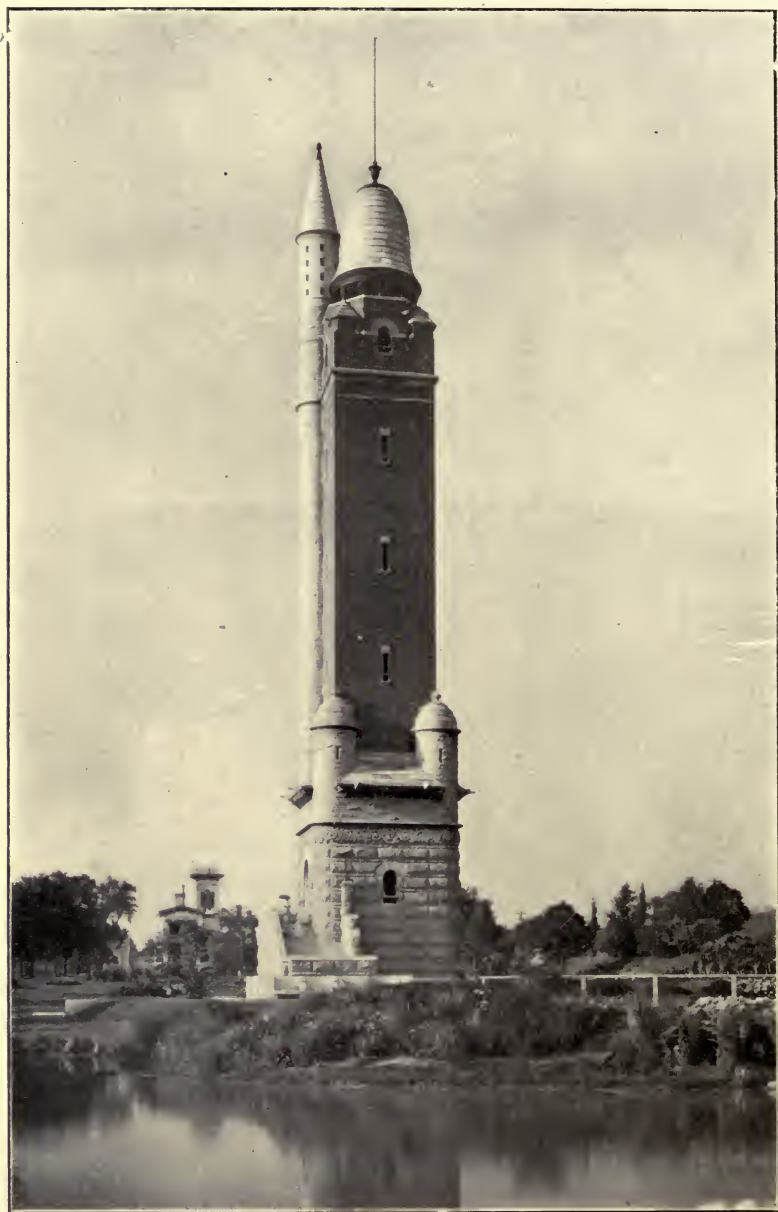
FIG. 53.—ST. LOUIS WATER-TOWER.
