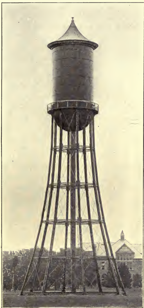
FIG. 54.—AMES, IOWA, STEEL WATER-TOWER.
