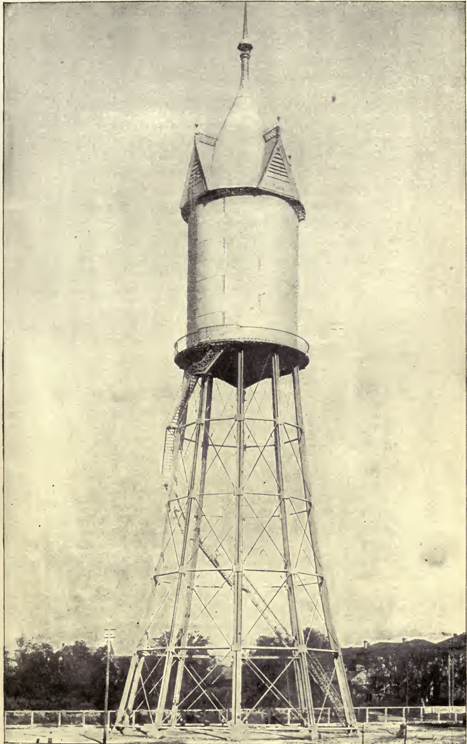
FIG. 2.—JACKSONVILLE, FLA., WATER-TOWER. R. D. Wood & Co., Philadelphia, builders.
