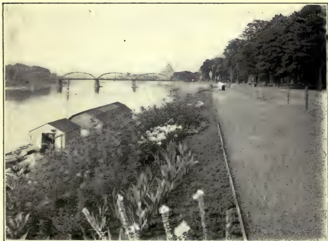
THE SAME RIVERFRONT AFTER IMPROVEMENT A forceful example for other towns and cities.
