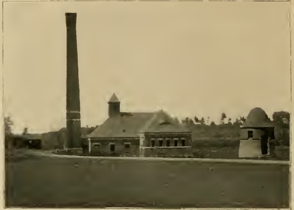
SEWERAGE PUMPING STATION
