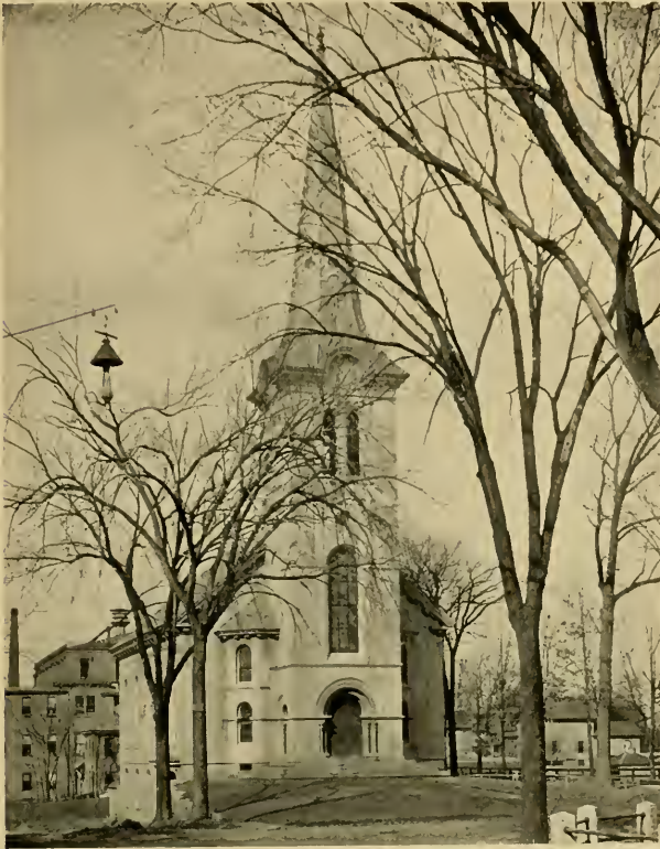
Park Street Baptist Church, South Framingham
