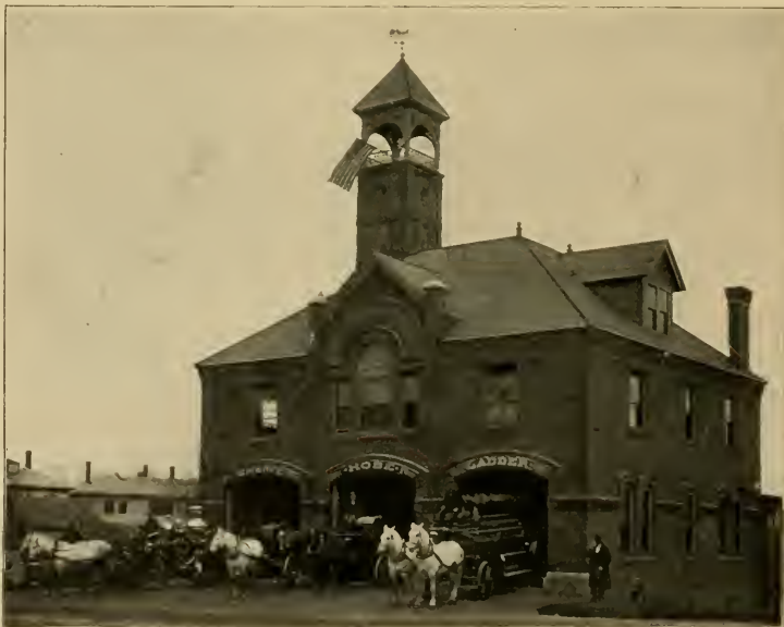
Central Fire Station, Hollis Street, South Framingham
