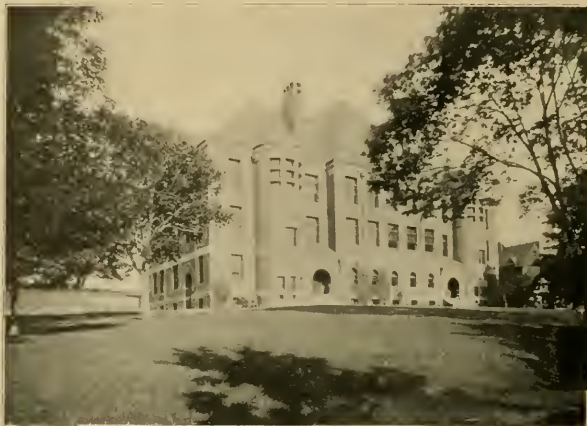
State Normal School, Framingham Centre
