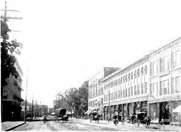
Concord Street, Looking South
