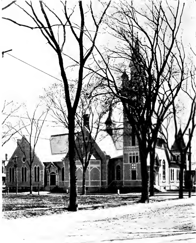
Grace Congregational Church. South Framingham
