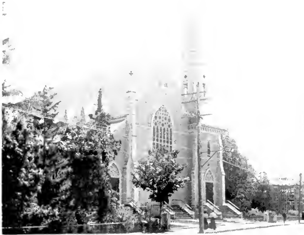
St. Stephen's Catholic Church, South Framingham
