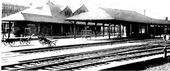
B & A Railroad Station, South Framingham
