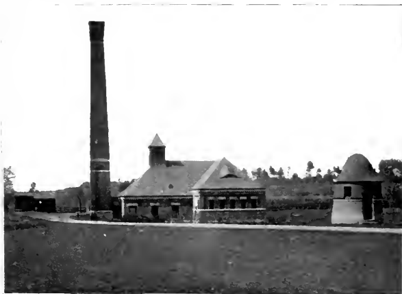
SEWERAGE PUMPING STATION
