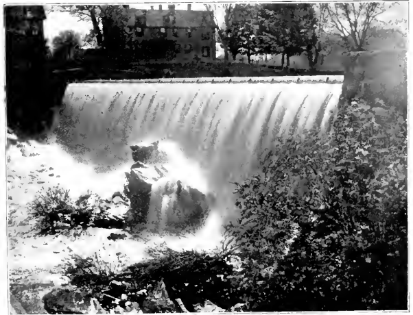
Dam at Saxonville Mills
