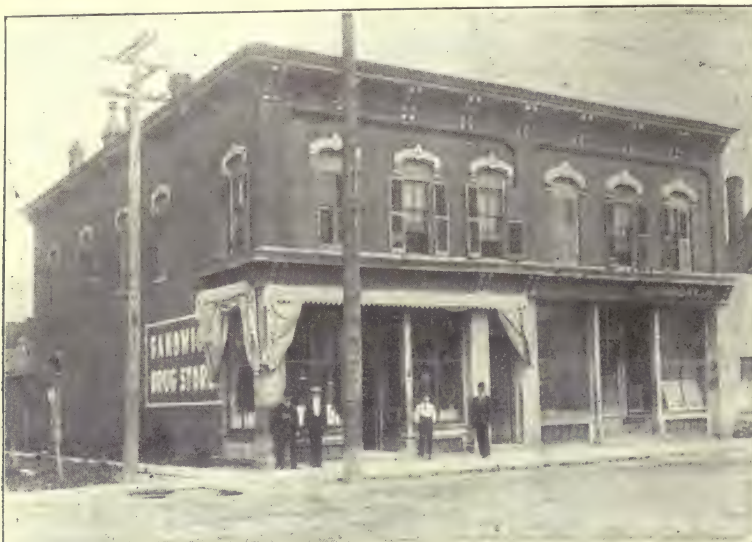
THE GIRARDOT BUILDING.
