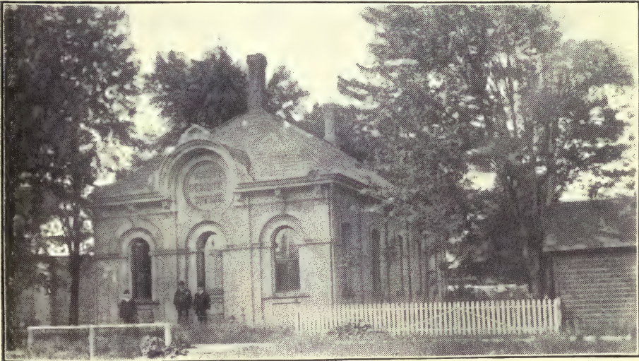
ESSEX COUNTY REGISTRY OFFICE, SANDWICH, ONT.
