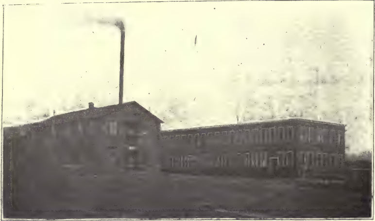
THE J. H. BISHOP FUR COMPANY'S BUILDINGS, RUSSELL ST., SANDWICH. W. J. Burns, resident manager.
