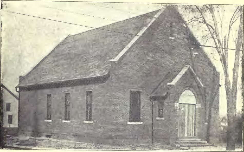
ST. JOHN'S CHURCH HOUSE, Northwest corner of Huron and Bedford Streets. Built in 1906.
