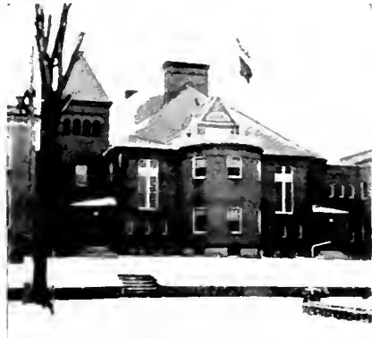
From a photograph Kindness F. E. Wing, Esq. HIGH SCHOOL BUILDING, ATHOL, MASSACHUSETTS,
