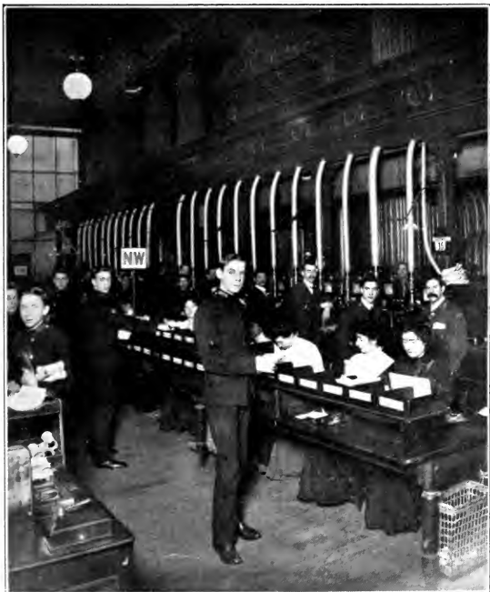
THIS ILLUSTRATION SHOWS THE PNEUMATIC TUBES THROUGH WHICH TELEGRAMS SENT FROM CENTRAL LONDON POST OFFICES ARE RECEIVED AT THE G.P.O. TO BE DESPATCHED BY TELEGRAPHISTS OVER THE WIRES.
