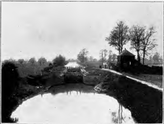
CANAL WITH LOCK. THE WATER BEYOND THE LOCK IS AT A HIGHER LEVEL THAN THAT NEARER THE SPECTATOR
