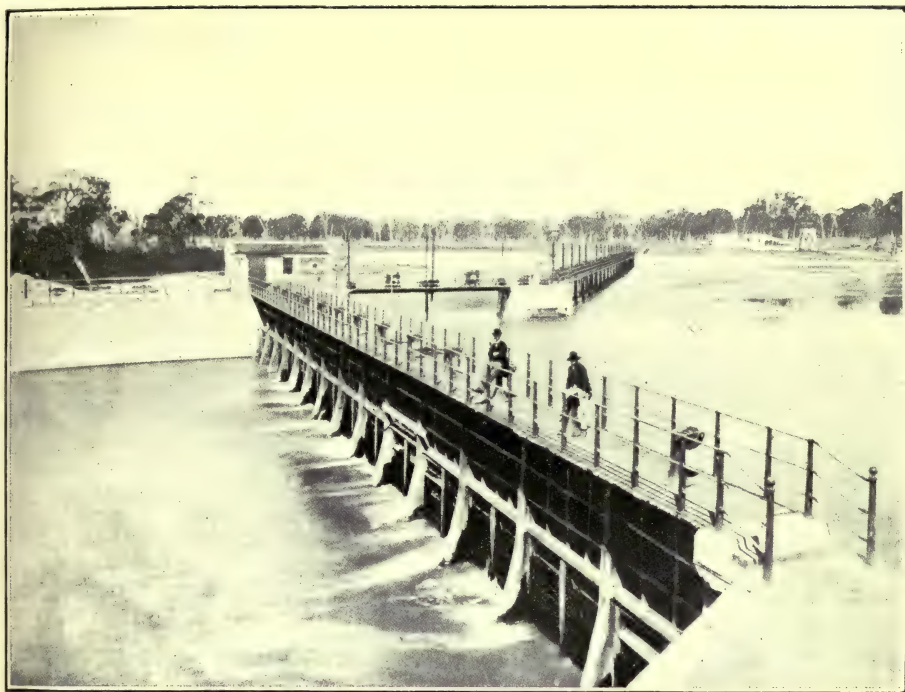
IRRIGATION WORKS IN VICTORIA. WEIR AT GOULBURN.
