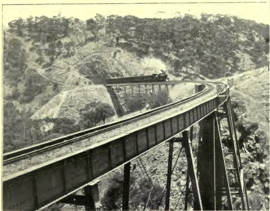
VIADUCT AT MITCHAM ON THE ADELAIDE-MELBOURNE RAILWAY.
