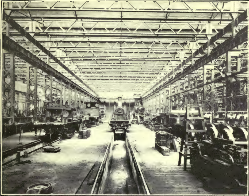
VIEW IN THE MIDLAND JUNCTION LOCOMOTIVE ERECTING SHOP, WESTERN AUSTRALIA.
