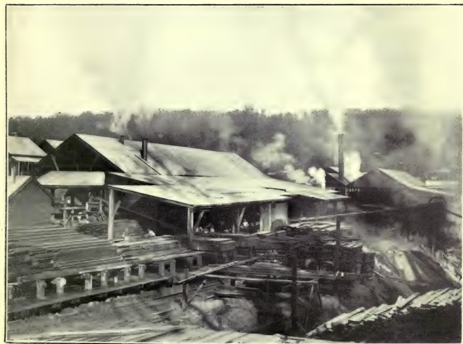
THE MORNINGTON TIMBER MILLS OF THE KARRI AND JARRAH CO.
