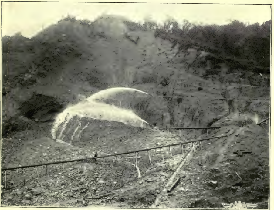
HYDRAULIC GOLD MINING IN NEW ZEALAND.
