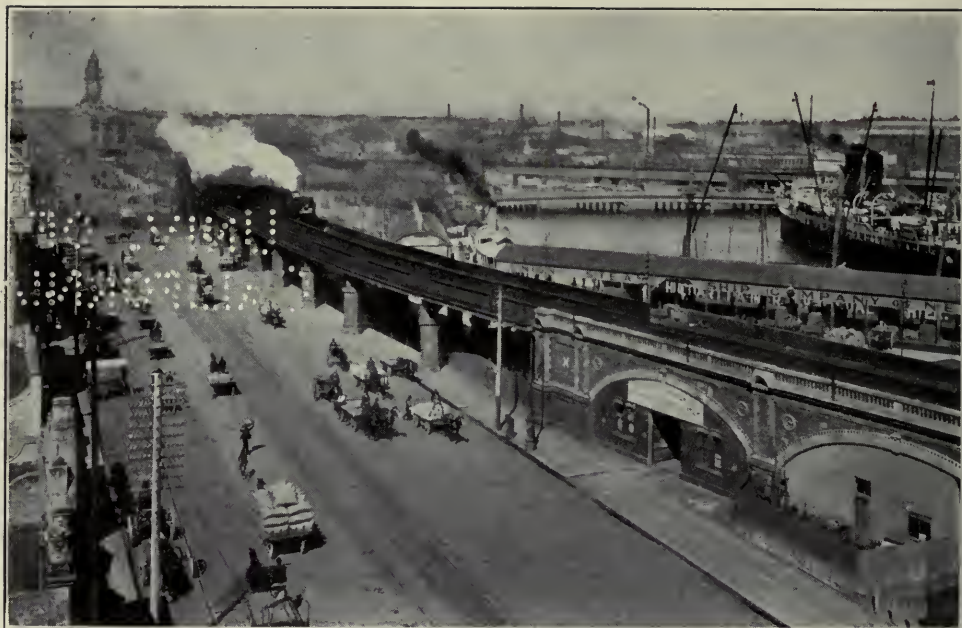
The railway viaduct in Melbourne
