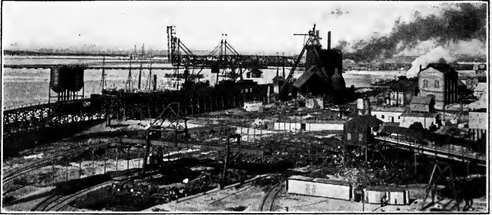
A steel plant at Newcastle, New South Wales
