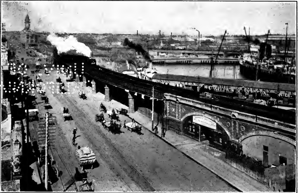
The railway viaduct in Melbourne
