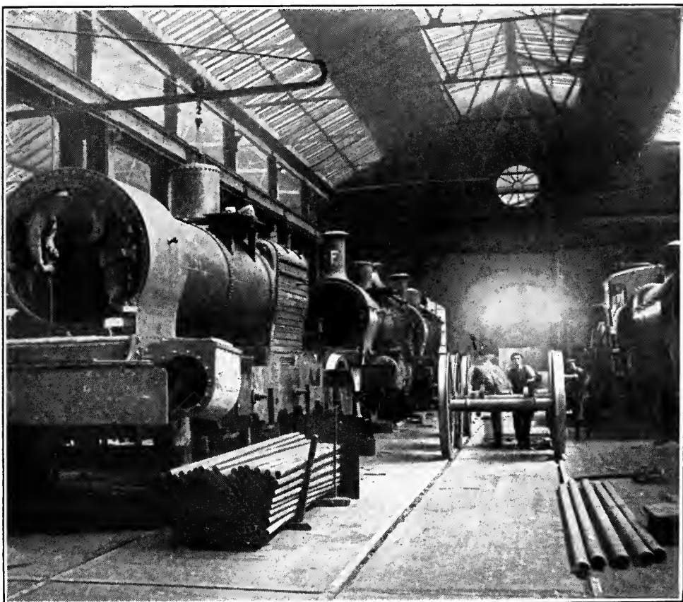
Government railroad shops at Williamstown, Victoria
