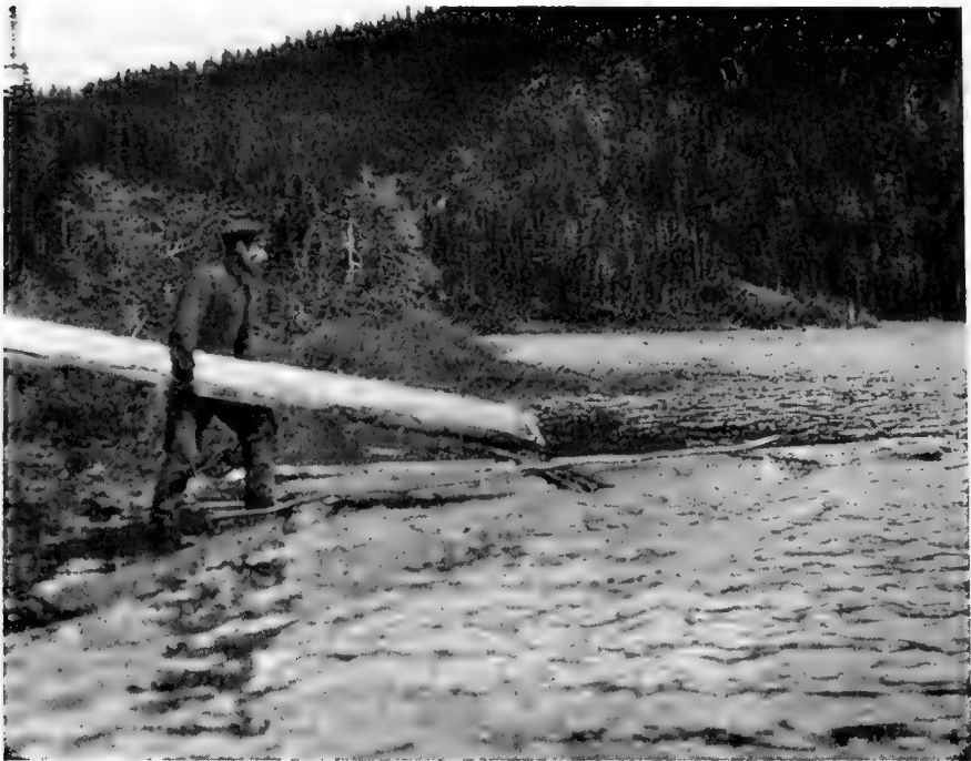
Constructing a Raft
