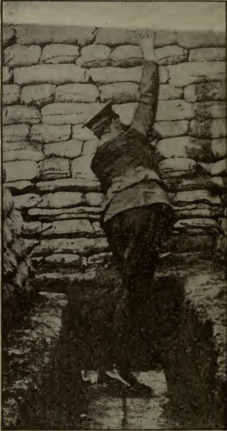
AFTER THROWING FROM A DEEP TRENCH.
