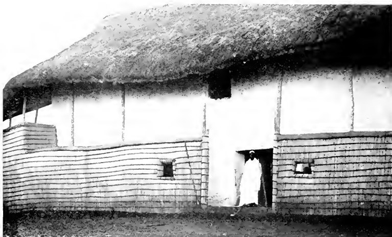
DAUDI KASAGAMA, OUTSIDE HIS BRICK PALACE, THE ONLY TWO-STORIED BUILDING IN TORO.
