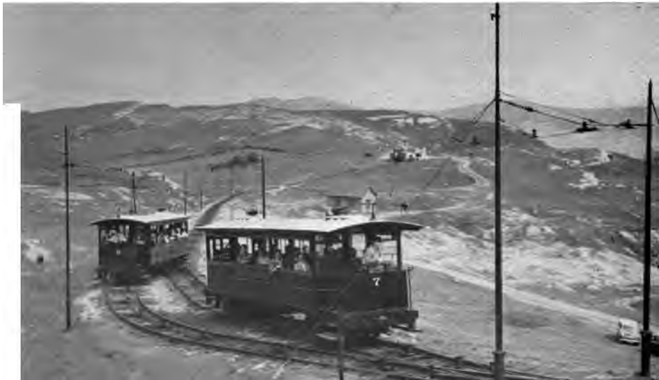
(Below) Cars passing on the upper section of the Great Orme Railway, with the winding station in the background. The overhead wire is for communication only. (Photos: English Electric Co. Ltd.)
