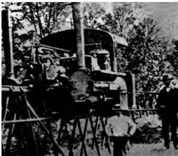
(Top) Locomotive on the Feurs-Panissières Lartigue monorail line in France (1894).
