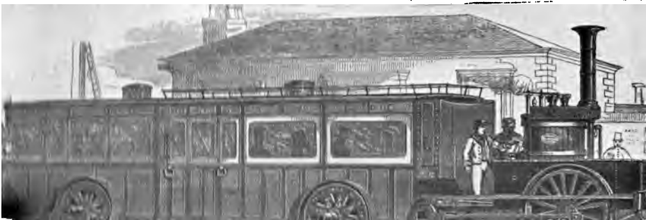
(Below) The "Fair-Field" railway steam carriage—one of the first self-propelled railcars.
