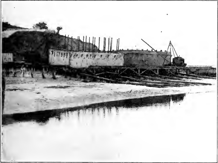
Smaller Caissons Nos. 2 and 3 ready for launching at Sillery.
