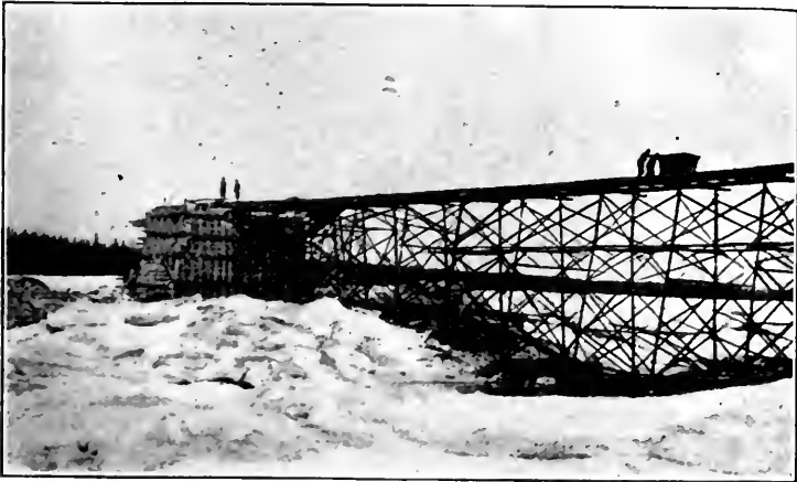
Fig. 2:—Pier 2 under construction.
