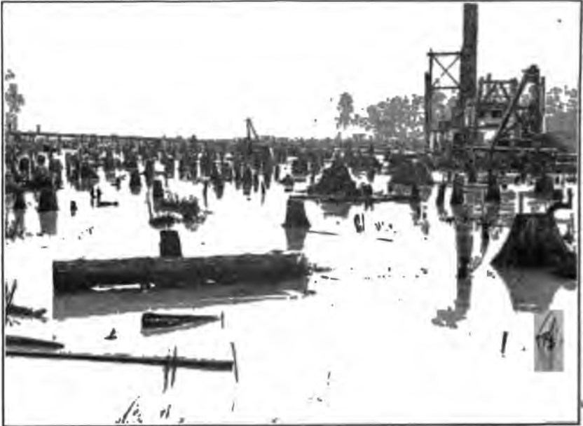
FIG. 3 CHARACTER OF EXCAVATION ENCOUNTERED
