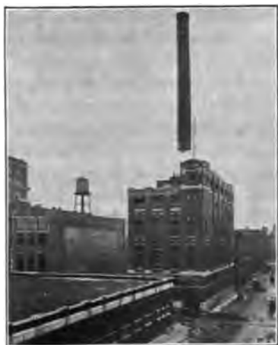
Congress Street Plant
