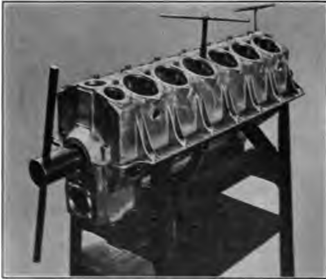
FIG. 13. LIBERTY MOTOR CRANKCASE ASSEMBLED
