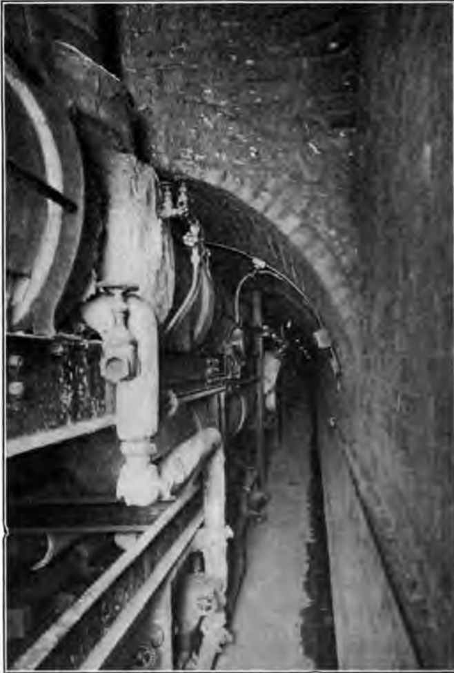
FIG. 9 TUNNEL CONSTRUCTION FOR STEAM LINES
