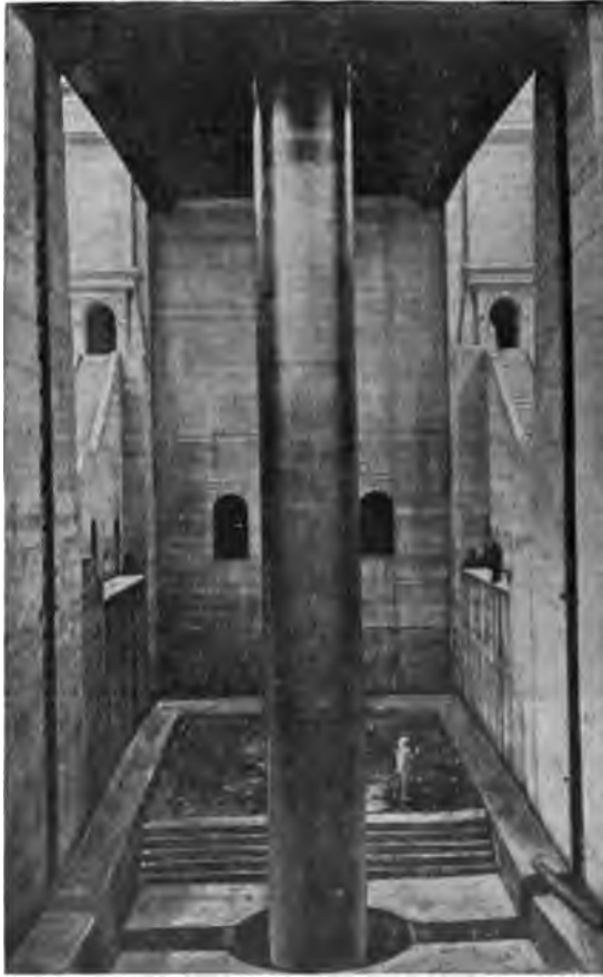
FIG. 2 ONE OF THE PLUNGERS OF THE PETERBOROUGH LOCK
