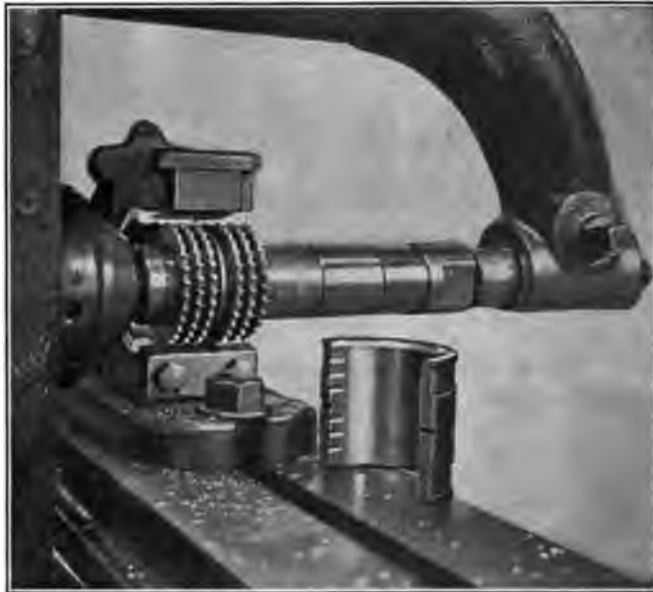
FIG. 11 METHOD OF CUTTING OIL GROOVES — OPERATION 20
