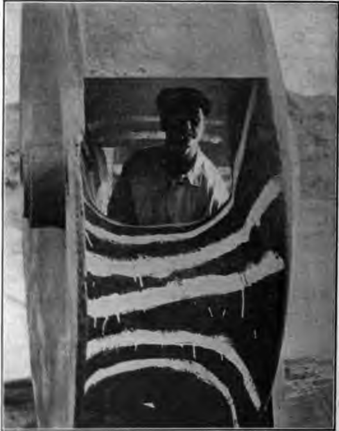
FIG. 10. VIEW SHOWING THE LARGE PASSAGEWAYS OF THE IMPELLER DESIGNED BY A. B. WOOD
