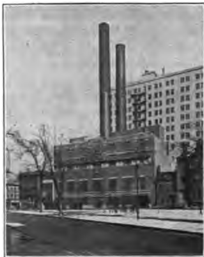
Park Place Plant
