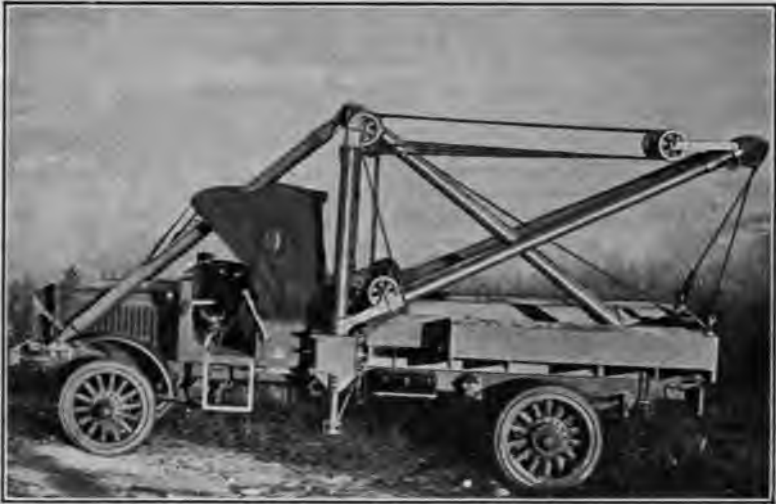
FIG. 10 A SPECIAL TYPE OF WRECKING APPARATUS MOUNTED ON A "B" TRUCK
