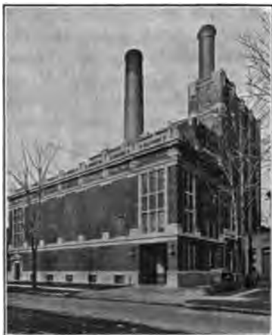
Willis Avenue Plant
