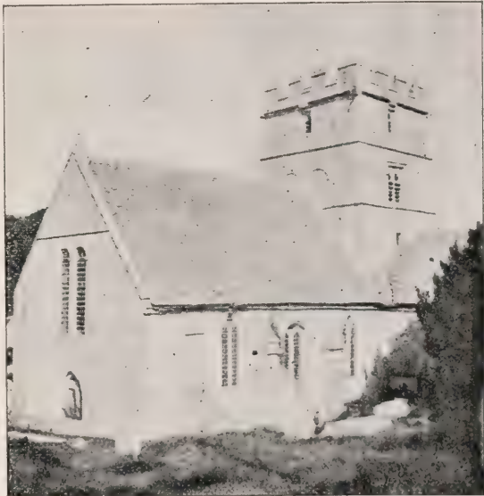
VIEW OF CHURCH FROM S.W.
