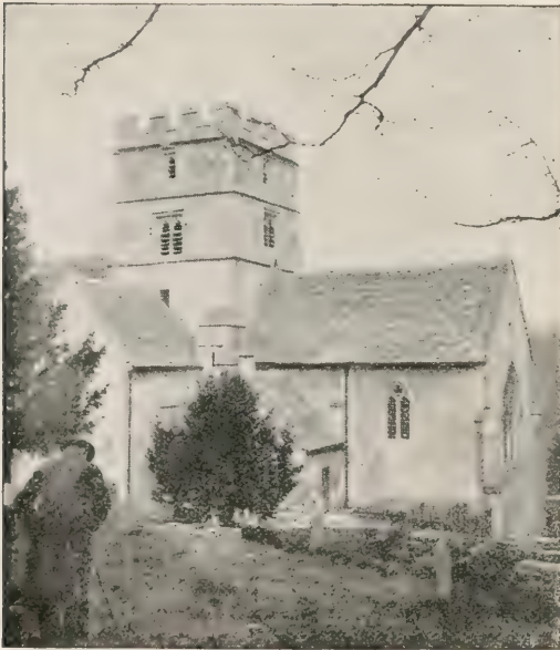
VIEW OF CHURCH FROM S.E.
