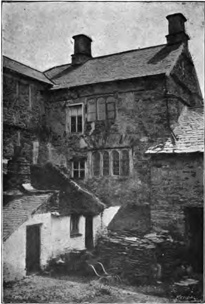
CAWMIRE HALL. (North side of Pele Tower.)
