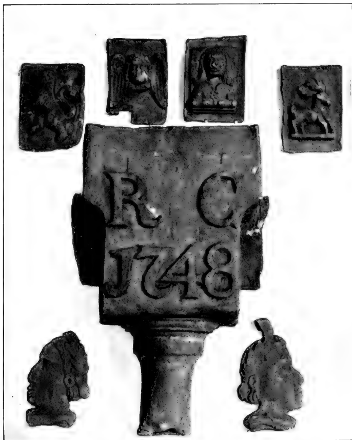
LEADWORK (RAINBOX AND LUGS) FROM OLD BLUE BELL INN, ST. MICHAEL'S STREET, DUMFRIES.
