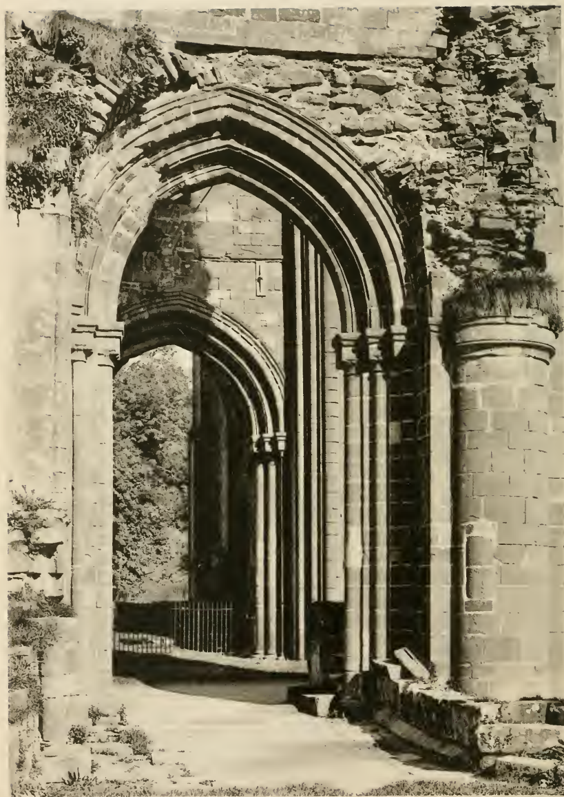
ARCH AND RESPOND AT EAST END OF NORTH AISLE.
