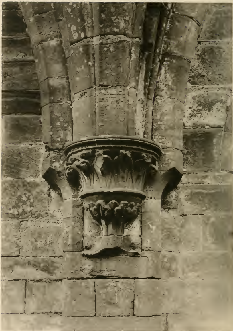
VAULTING CORBEL IN THE DORTER SUB-VAULT.
