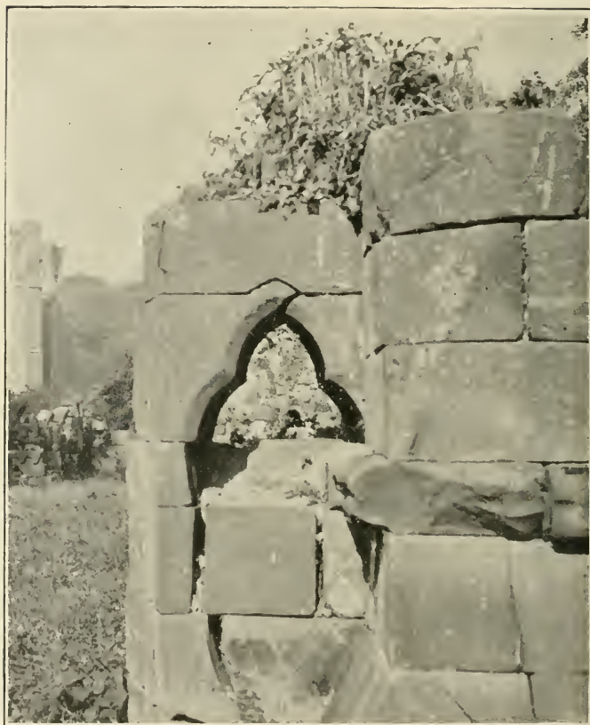
TREFOILED OPENING IN THE SOUTH WALL OF THE OLD INFIRMARY HALL.
