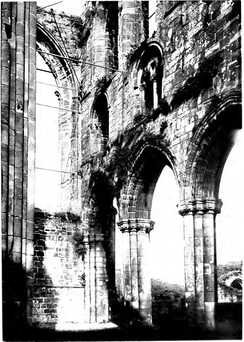
EAST SIDE OF THE NORTH TRANSEPT.
