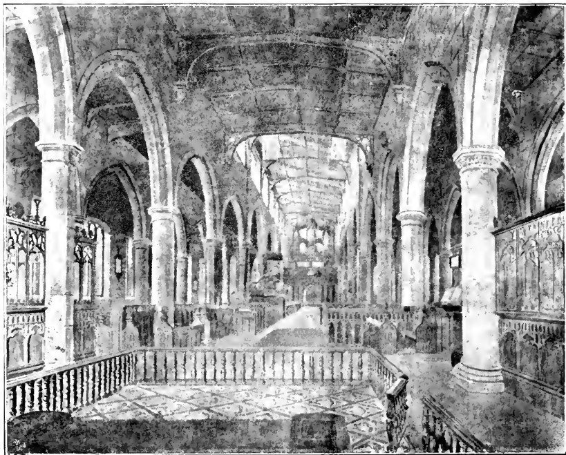
INTERIOR LOOKING WEST, 1830.
