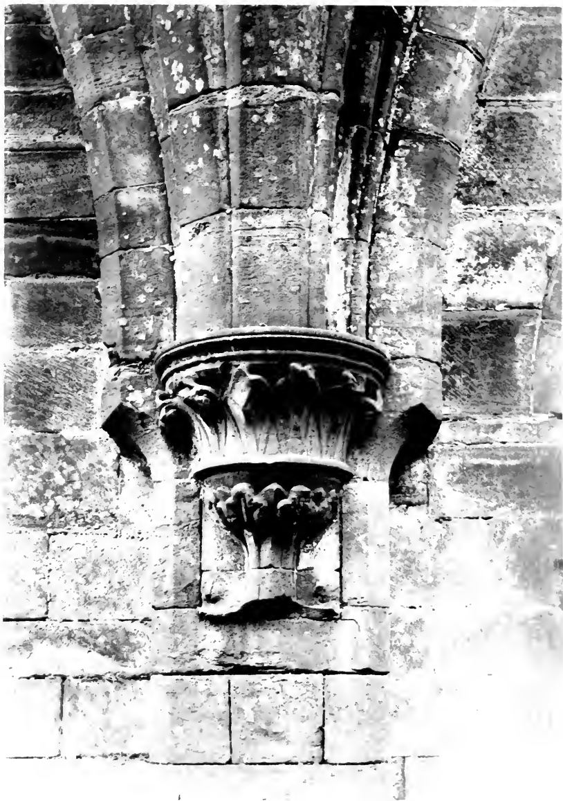
VAULTING CORBEL IN THE DORTER SUB-VAULT.
