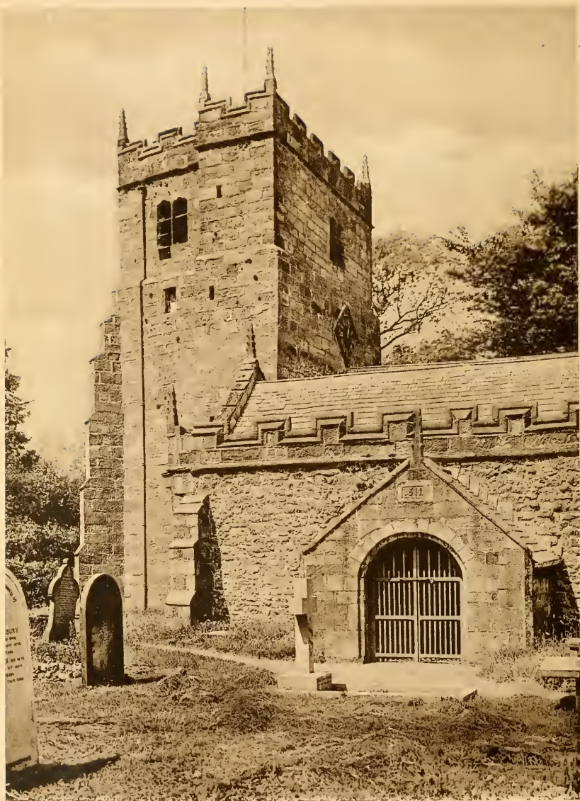
St. MICHAEL'S: Tower and South Porch.
