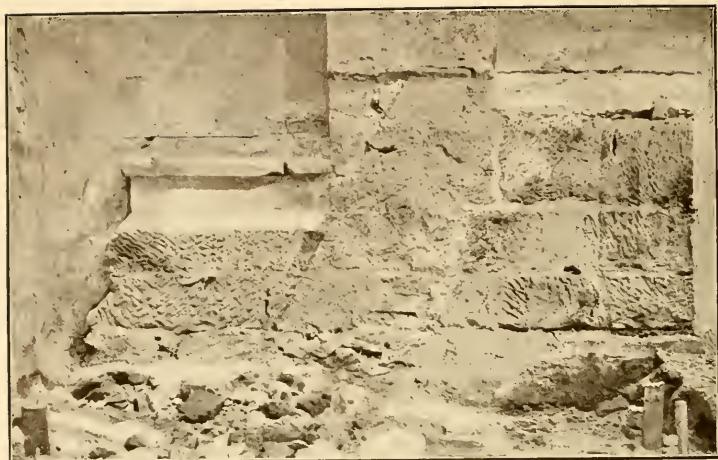
LOWER PART OF EAST WALL, NORTH AISLE, Showing how it was hacked away
