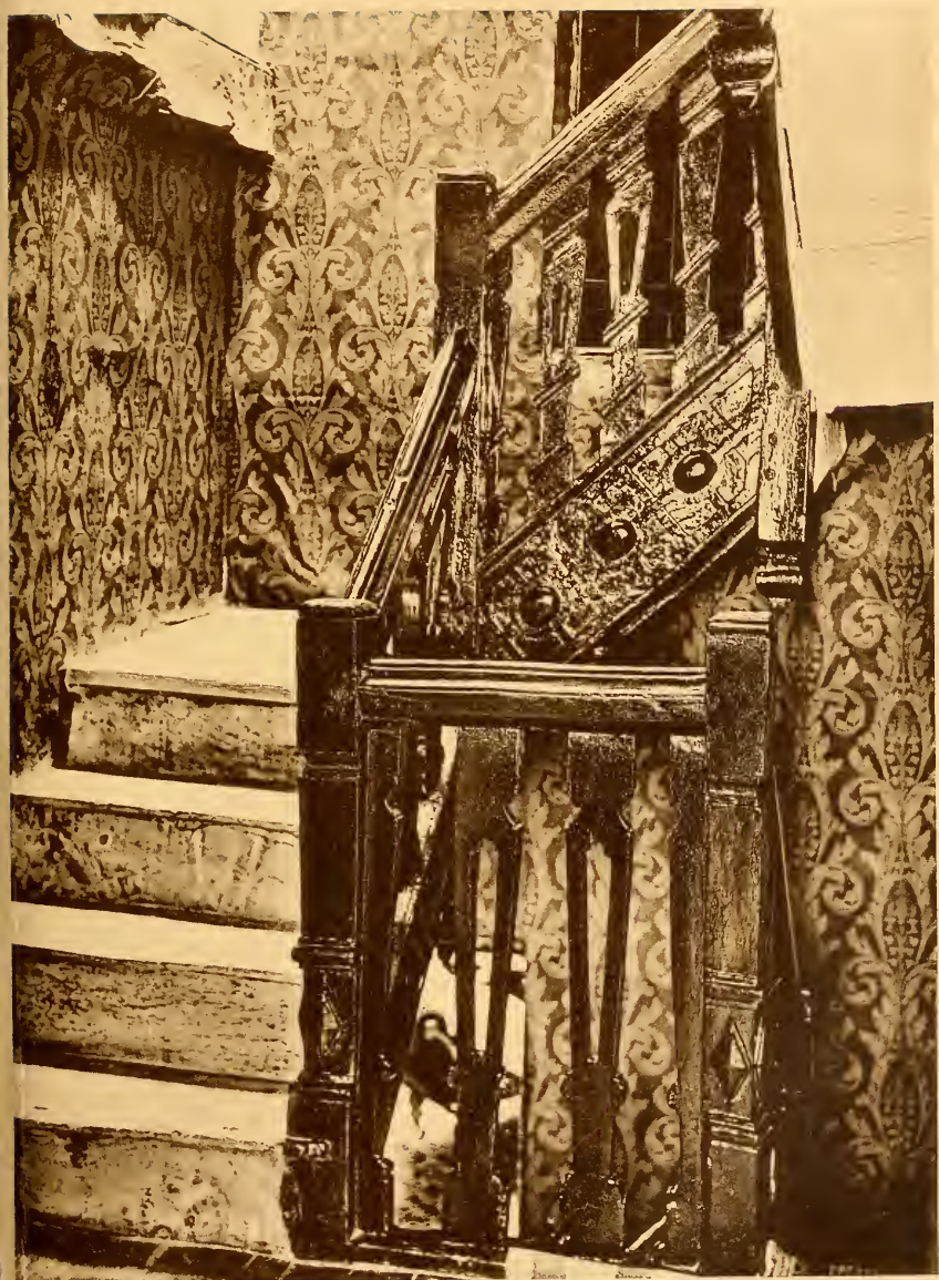
STAIRCASE, SHOTWICK HALL.
