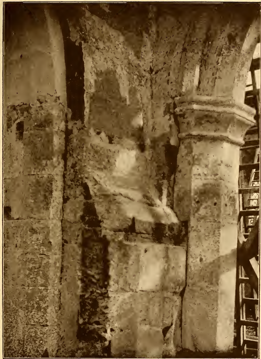
THE EAST PIER OF NAVE ARCADE,
