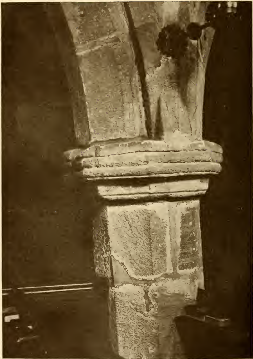
ST. MICHAEL'S: PIER IN NORTH ARCADE
