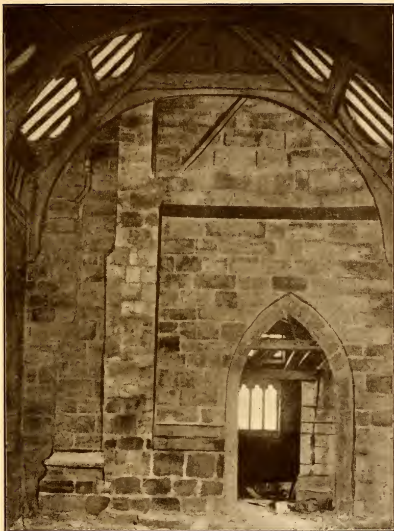
NORTH AISLE: EAST WALL AND BASE OF TOWER
