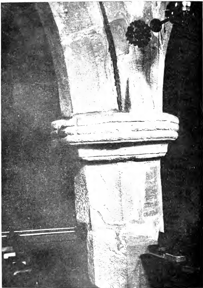
ST. MICHAEL'S: PIER IN NORTH ARCADE
