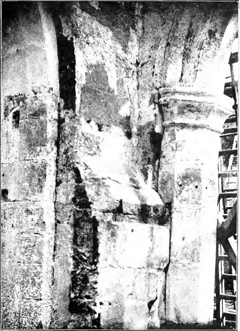
THE EAST PIER OF NAVE ARCADE,
