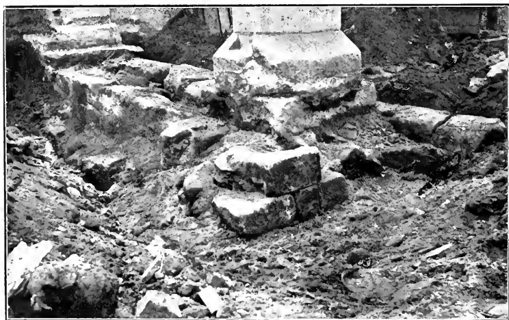
REMAINS OF NORMAN WEST WALL AND EARLY ENGLISH NORTH WALL UNCOVERED
