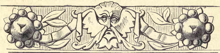
Cornice at No. 18, Bishopsgate Street Without.
