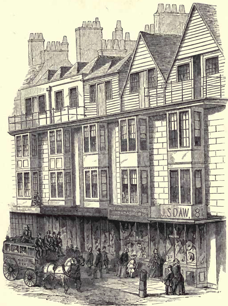
GROUP OF ELIZABETHAN HOUSES, Nos. 81—85, BISHOPSGATE STREET WITHOUT, 1857.
