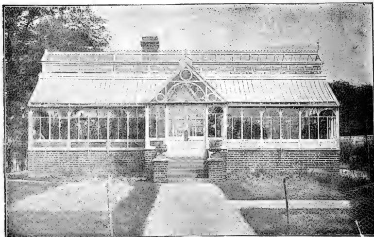
Conservatory Erected at Free Chase, Sussex.
