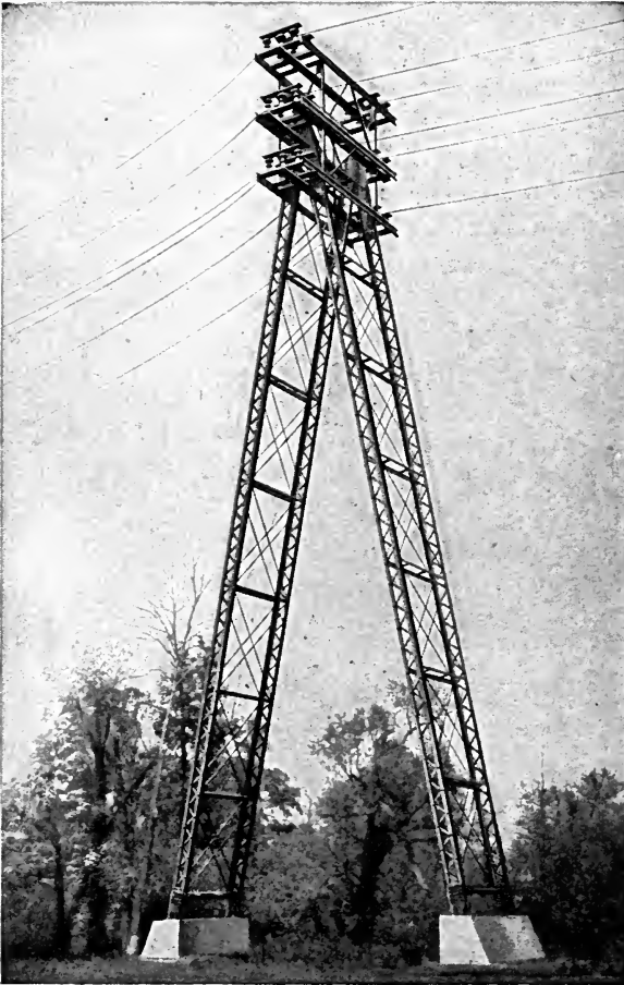
FIG. 96.—River crossing structure.
