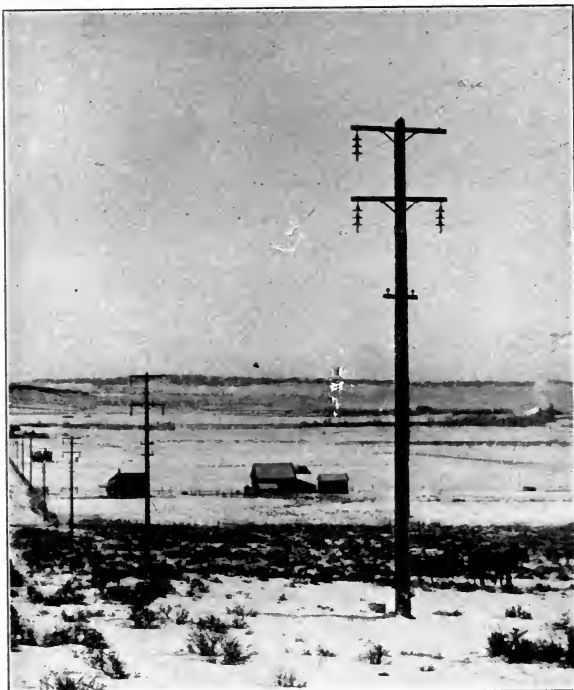
FIG. 13.—Madison River Power Company's long span wooden pole line.
