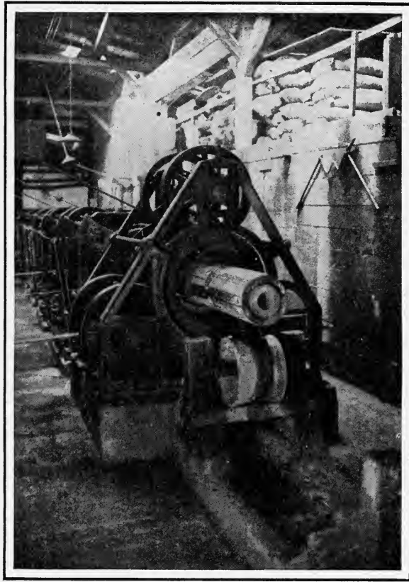
FIG. 82.—Machine used in molding centrifugal type concrete poles.
