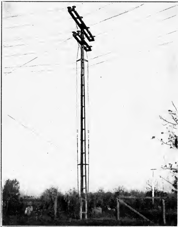
FIG. 150.—"Buck-stayed" or self-supporting pole.
