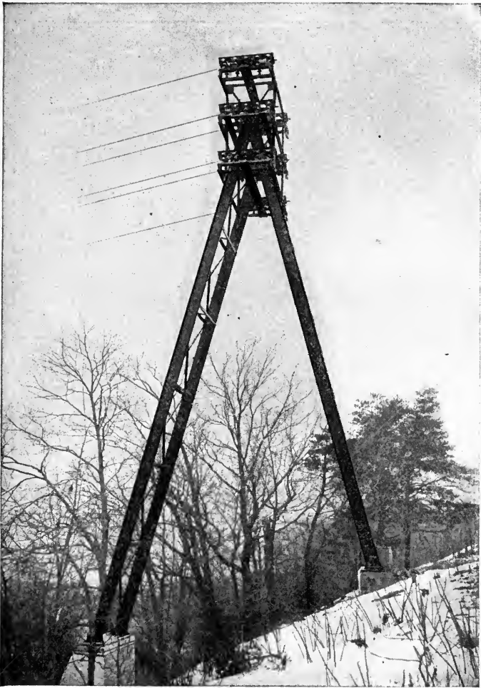
FIG. 95.—River crossing structure.
