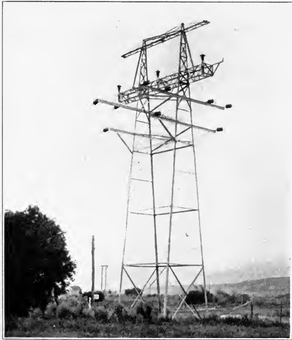
FIG. 115.—Joint tower at crossing of two high-tension lines.
