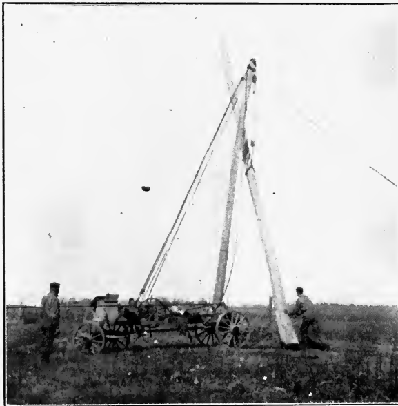
FIG. 40.—Erecting poles with gin wagon.
