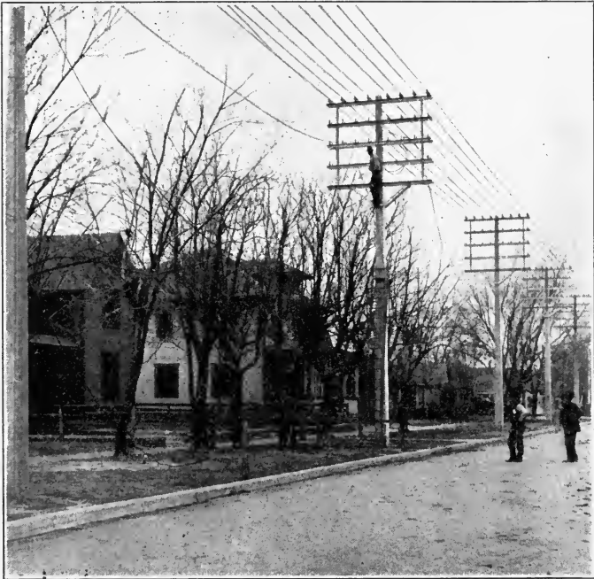
FIG. 86.—Oklahoma Gas & Electric Co.'s concrete poles.
