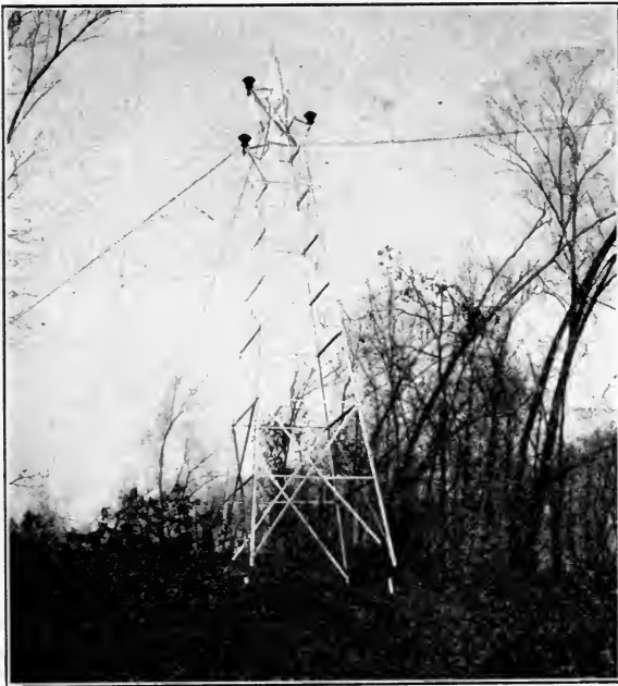
FIG. 74.—Raising tower with short shear pole.
