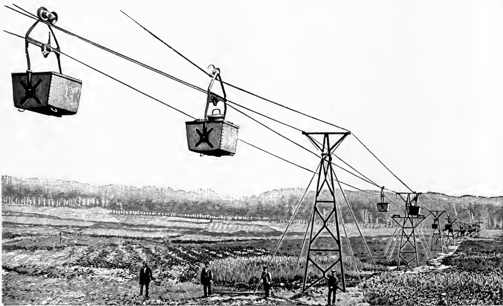
FIG. 4.—ILLUSTRATION OF AN "OTTO" ROPEWAY SHOWING LOADED BUCKETS ON ONE SIDE AND EMPTIES RETURNING ON THE OTHER.
