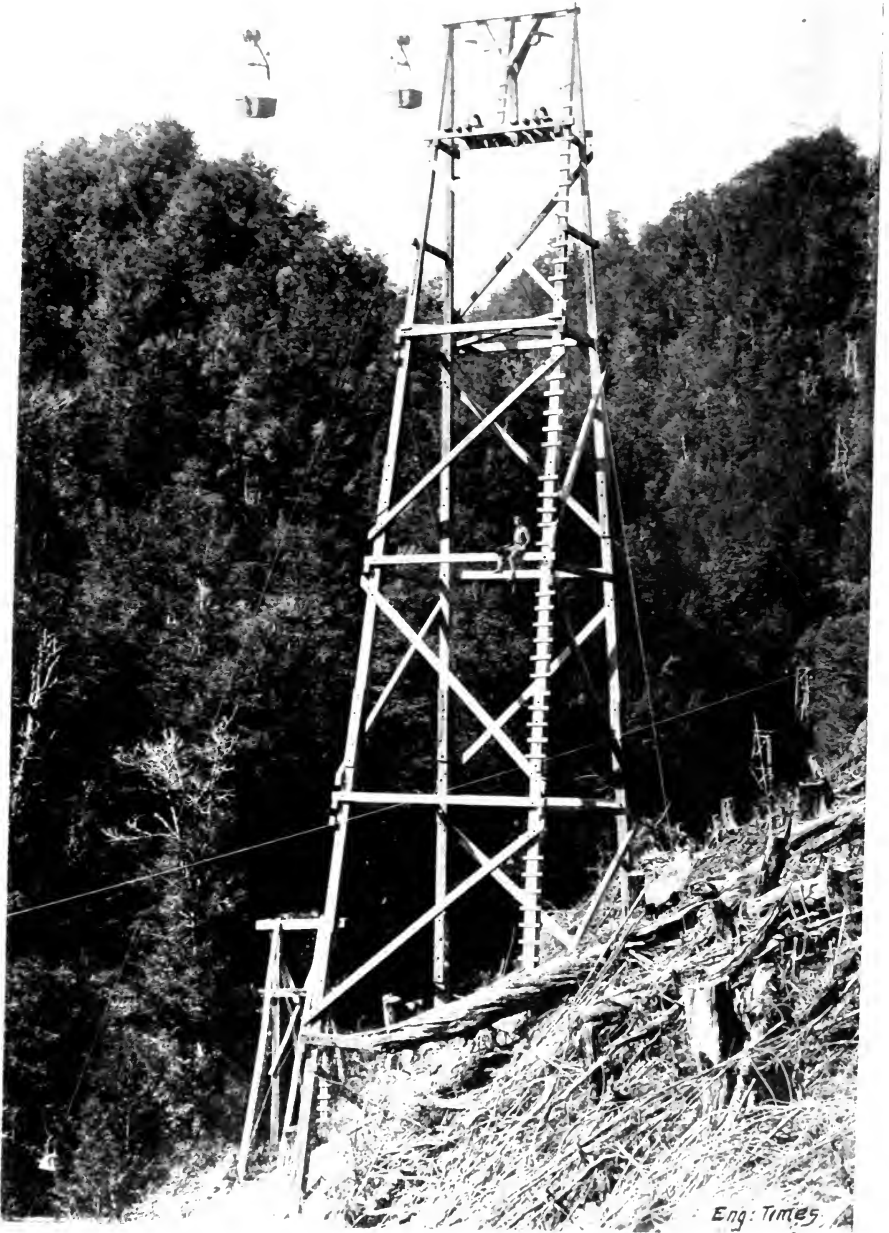
FIG. 4. EXAMPLE OF A WOODEN SUPPORT OF AN "OTTO" LINE IN NEW ZEALAND.
