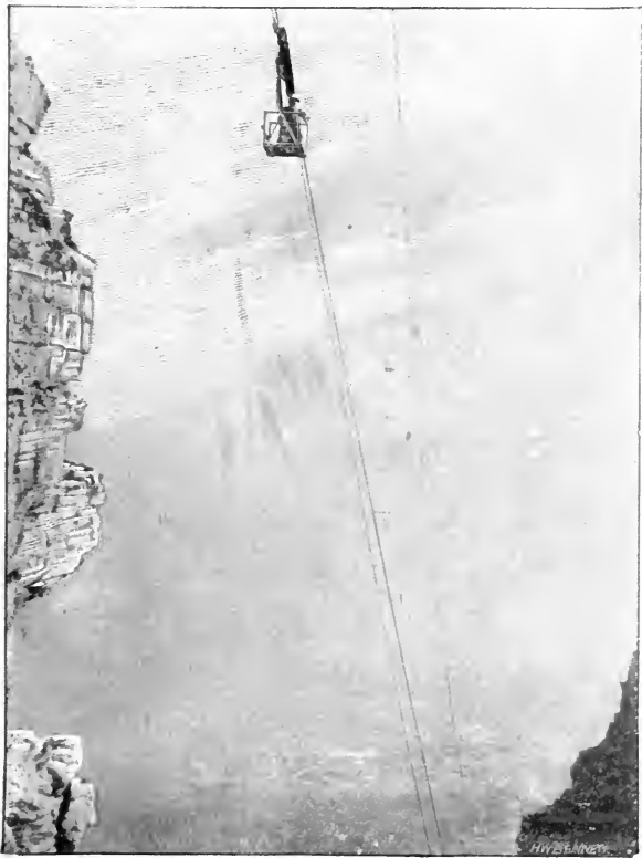
SECOND SPAN, SHOWING CARRIER IN TRANSIT.
