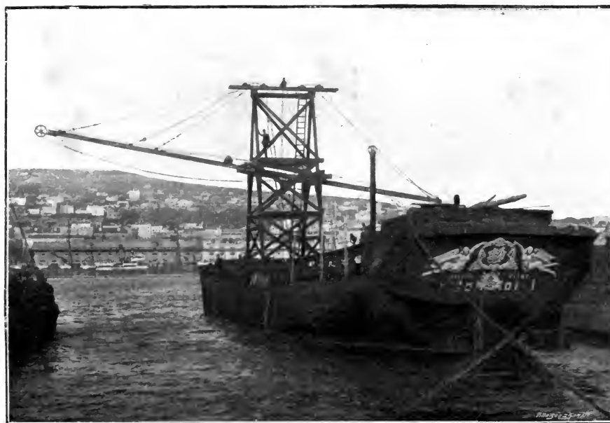
PORTABLE TOWER TRANSPORTER ON HULK.
