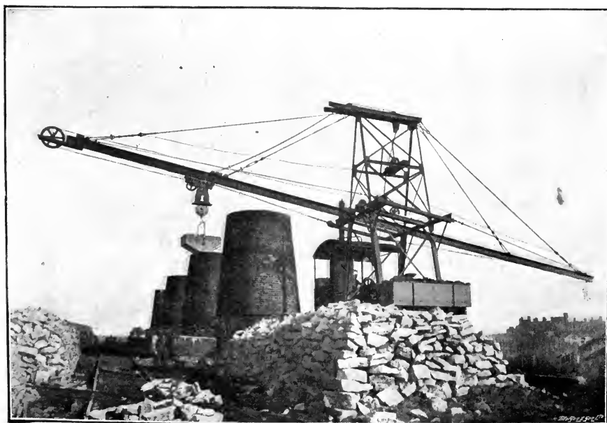
TRAVELLING TOWER TRANSPORTER. Serving Lime Kilns.
