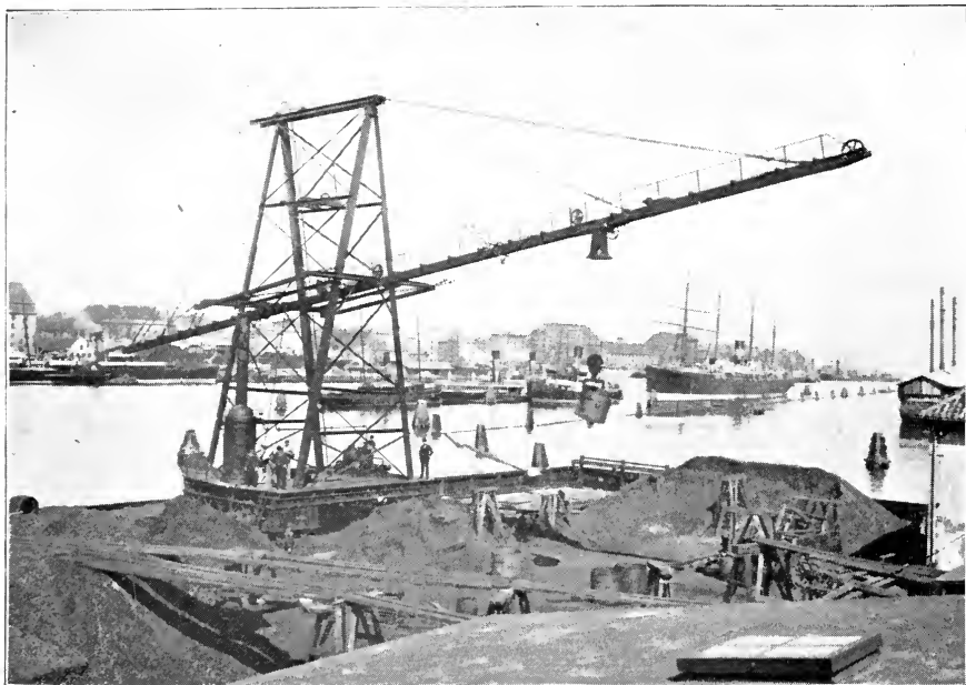
TRAVELLING TOWER TRANSPORTER. Discharging Coal, &c., from Steamers.
