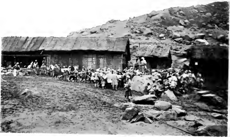
TOP STATION AT NEW RAPID.
