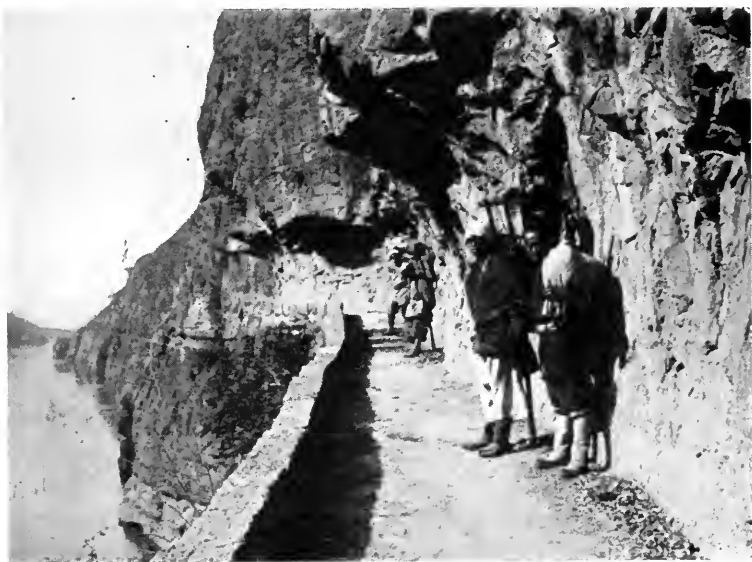
GALLERY CUT OUT OF SIDE OF CLIFF.
