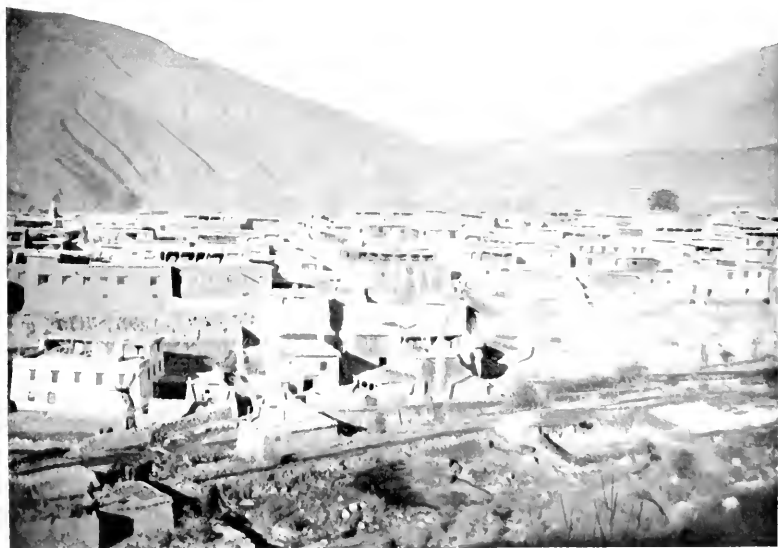
BATANG, LOOKING NORTH
