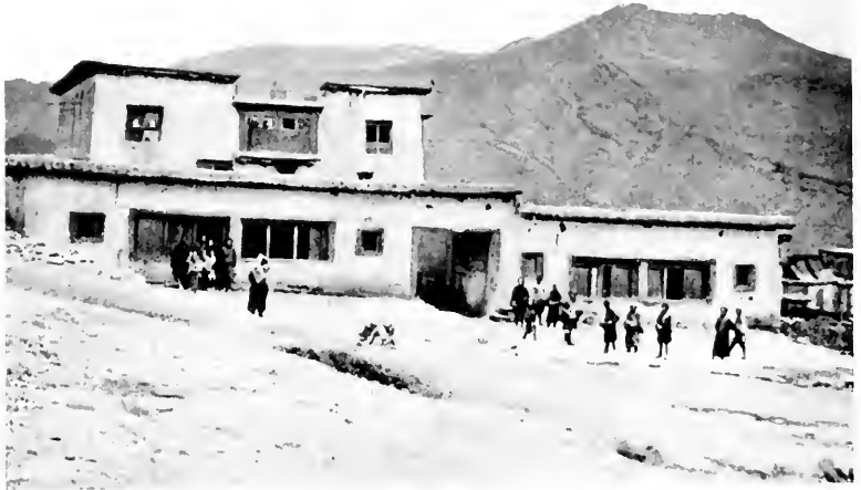
OFFICIAL'S HOUSE AT DRAYA JYAMDUN
