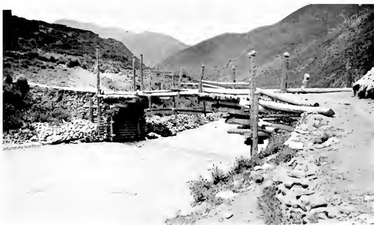
CANTILEVER BRIDGES IN EASTERN TIBET (MAIN ROAD TO LHASA, NEAR DRAYA)
