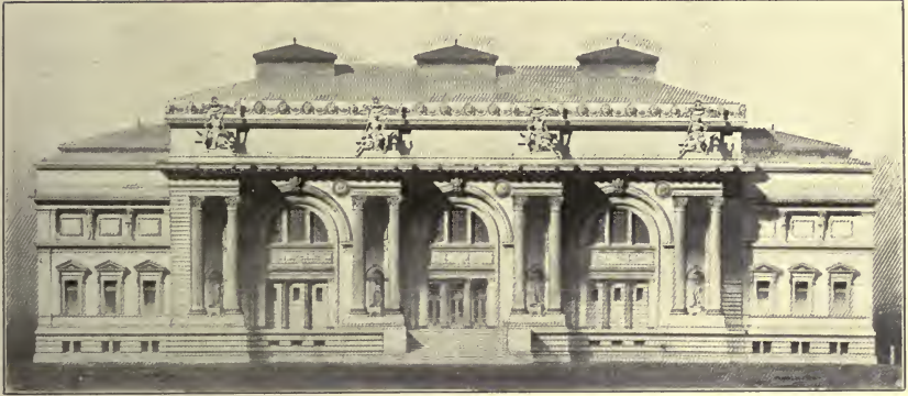
THE NEW WING.
