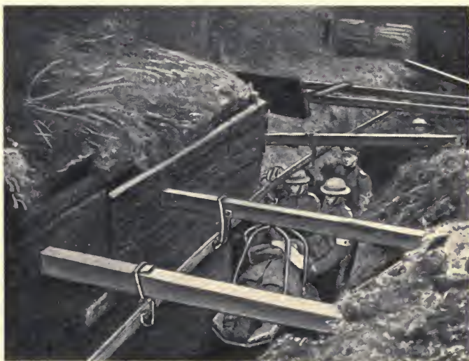
Fig. 6.—Overhead railway ambulance trolley (redrawn). (Kindness of the editor of the British Medical Journal and of Sir A. A. Bowlby, Bart. See Prefatory Note.)
