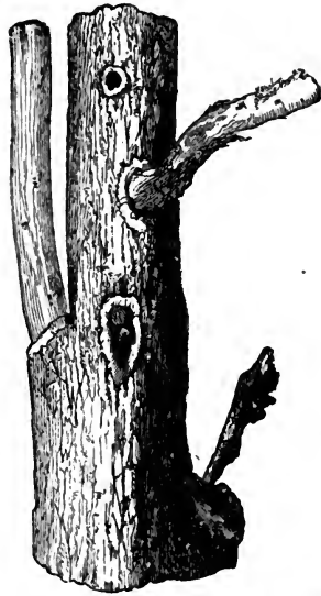
Fig. 3. — Portion of the trunk of an unpruned Oak ruined by the decay of its lower branches.
