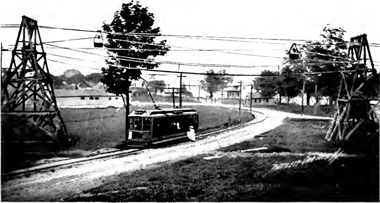
Guard Net on line of The Farnam-Cheshire Lime Co., Cheshire, Mass.
