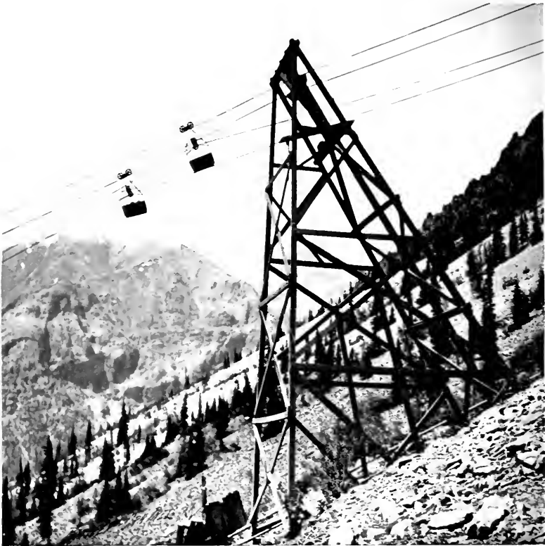
Fig. 27. Side Hill Support on line of the Old Hundred Mining Co., Howardsville, Col.
