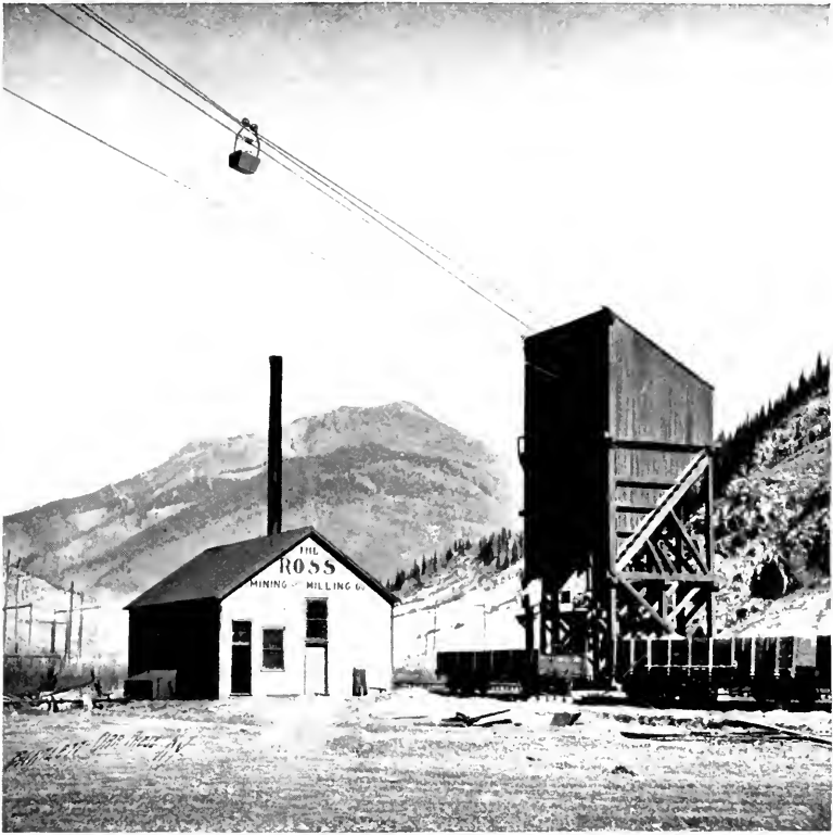
Double-Cable Reversible Tramway of The Ross Mining and Milling Co., Silverton, Col. View of Discharge Terminal.
