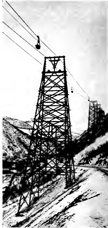
Fig. 25. Support 90 feet high, on line of The Yampa Smelting Co., Bingham, Utah.
