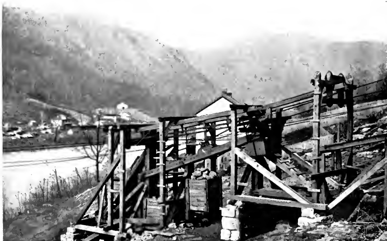
Fig. 30. Tension Station. Timber Structure.
