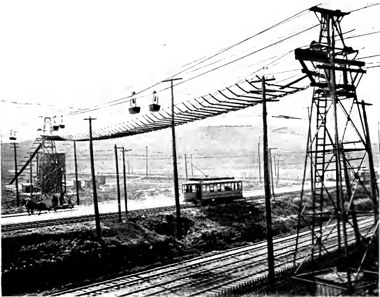
Guard Net on line of The Solvay Process Co., Solvay, N. Y.
