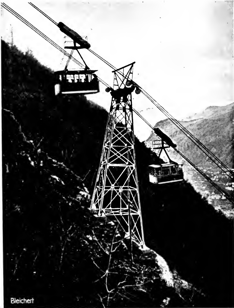
Passenger tramway in the Alps from the Eisack Valley to the summit of the Kohlererberg, in the Tyrol. Length, 5,420 feet. Difference in elevation between lower and upper terminal is 2,736 feet.
