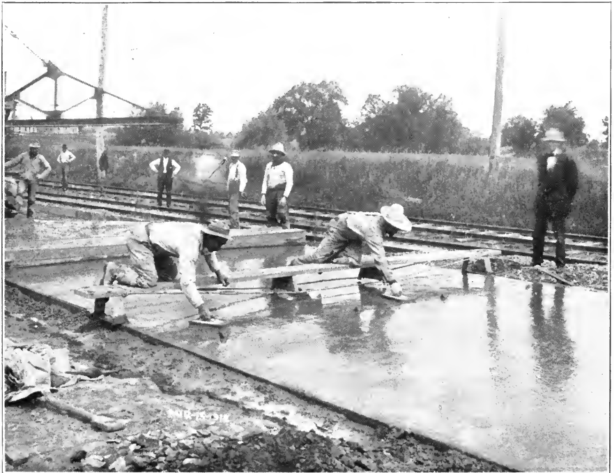
Finishing the Surface of Concrete Pavements.
