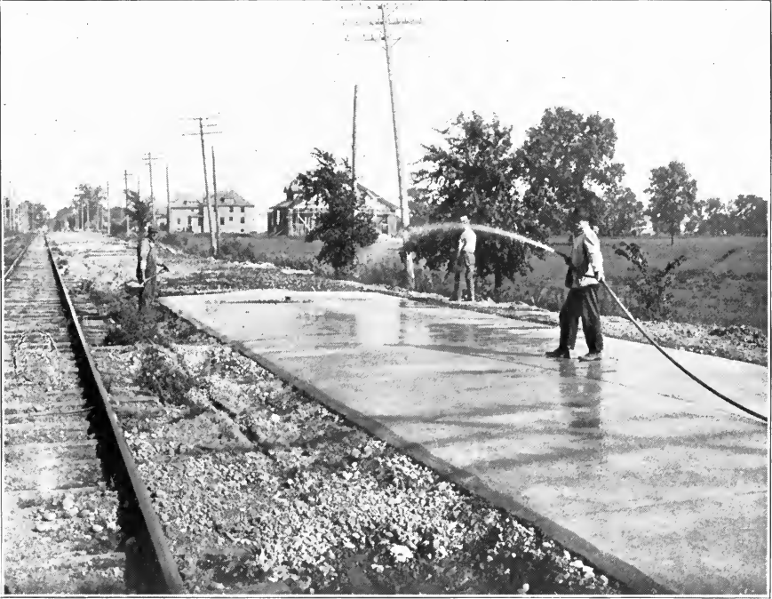
Concrete Pavement Protected with Dirt and Sprinkled Continuously for Several Days.
