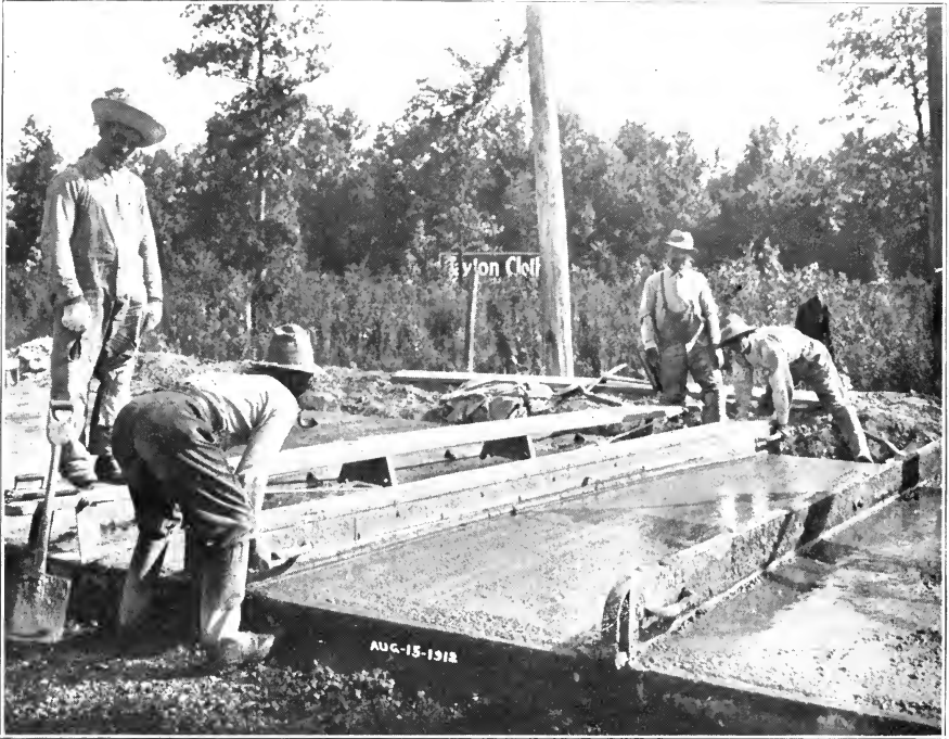
Striking Off Concrete Pavements
