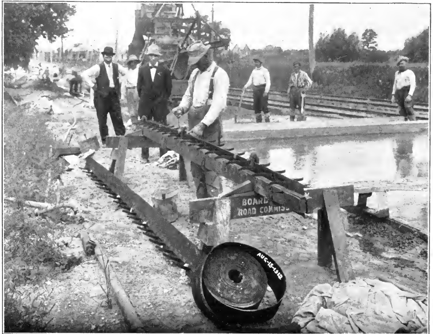
Preparing Steel Plate Expansion Joint Protection.
