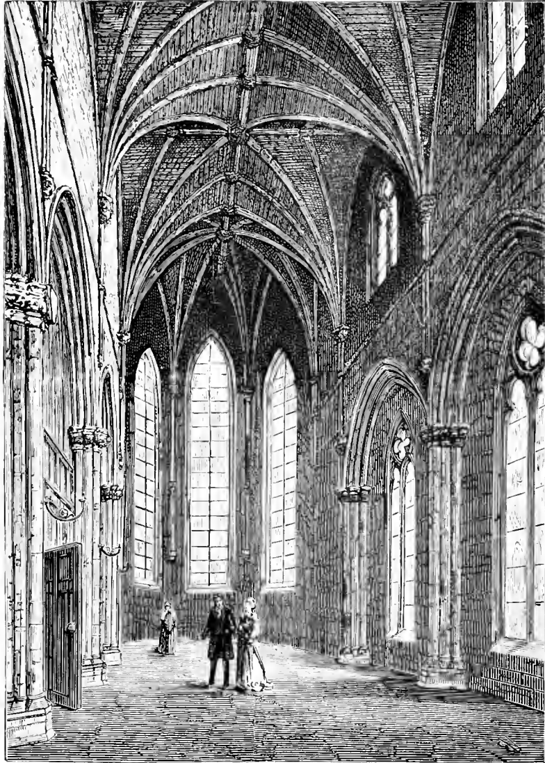
THE OLD APSE OF TRINITY COLLEGE CHURCH RESTORED.
