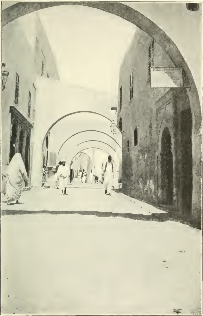
Pale blue-wash tinted many of the arches
